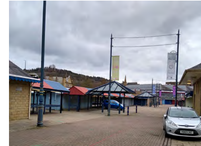
Figure 7.1.1 Cars are able to access the site despite bollards and gates being in place to prevent entry.
