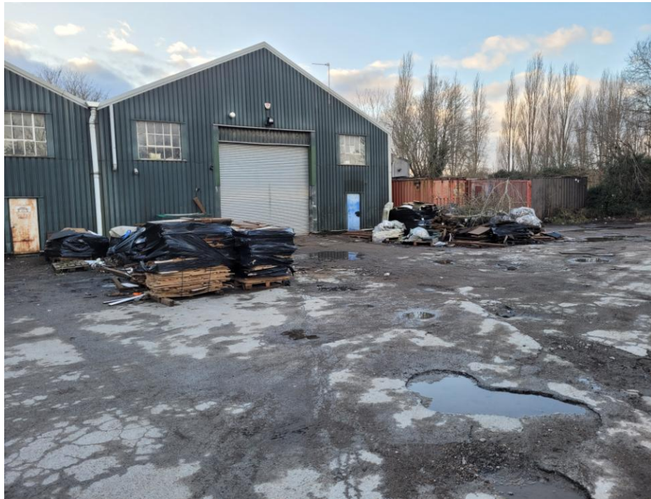
View of hardstanding, looking northwest towards works building
