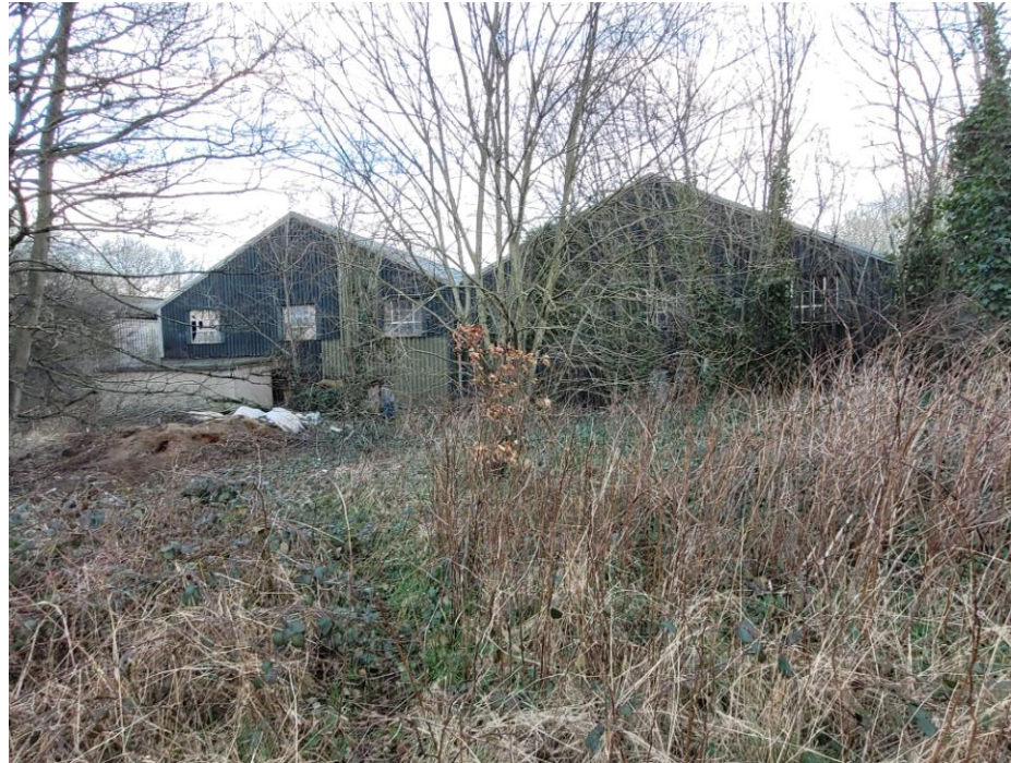
View of rear of buildings, looking northeast
