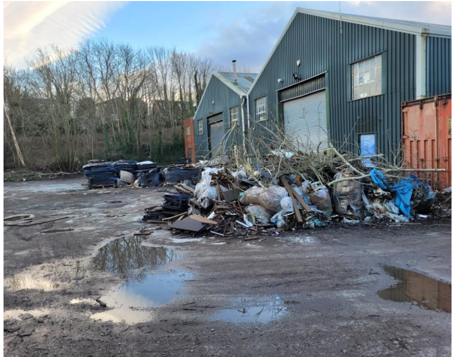
Waste material to front of works building
