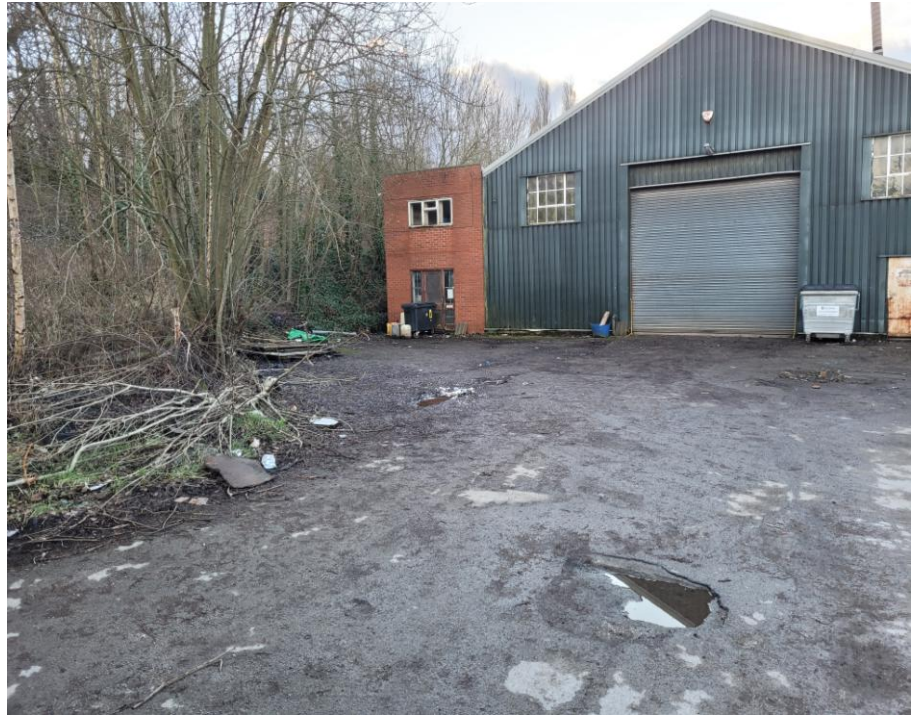
Main works building, looking southwest
