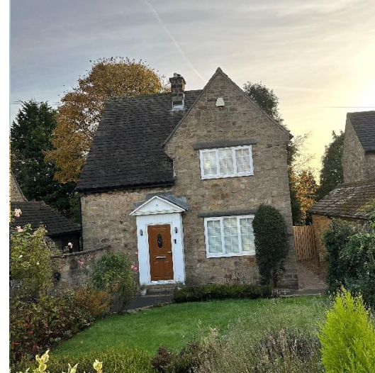
Approximate age: 1940s Key Features: Projecting porch with pointed pediment, rubble coursed stone, stone heads on front facing gable Material Palette: Yorkshire stone, timber projecting porch, stone roofing tile, white upvc windows
