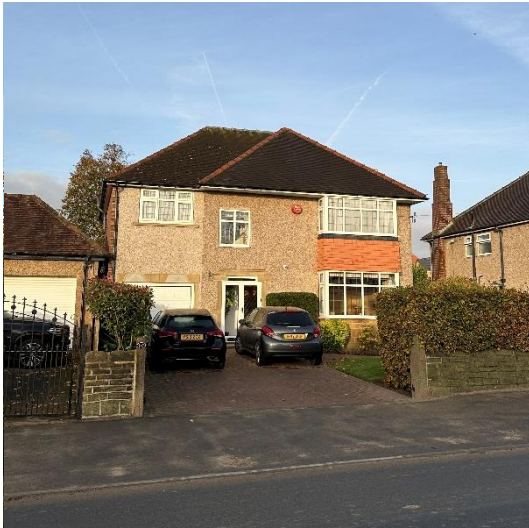
Approximate age: 1950s Key Features: Hipped roof with a two storey side extension, projecting bay window, distinctive ridge tiles Material Palette: Peddle dash, red brick, red walling tiles, white pvc windows and doors, grey roof tiles with red ridge tiles, stone heads
