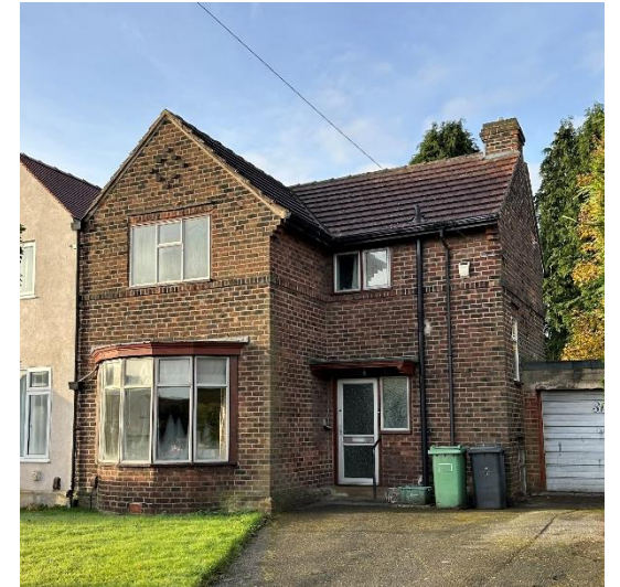
Approximate age: 1940s Key Features: Projecting brick string course, front bay window, projecting front gable Material Palette: Red brick, white pvc windows, red concrete roof tile
