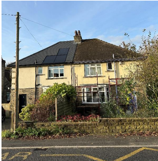
Approximate age: 1960s Key Features: Hipped roof, projecting bay windows, staggered stone quoins Material Palette: Yellow render, Yorkshire stone with extruded mortar, concrete roof tiles
