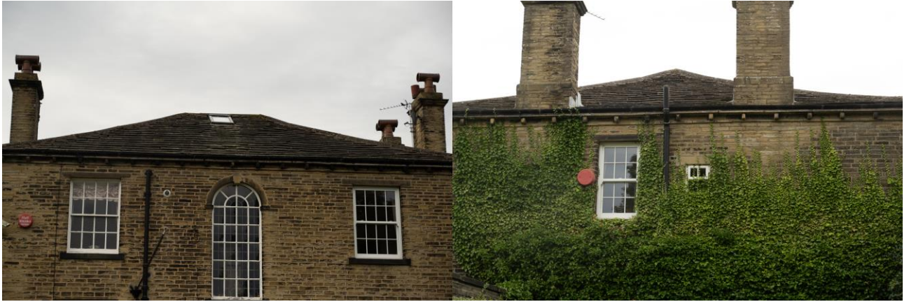
Photo 2: Illustrating roof section
