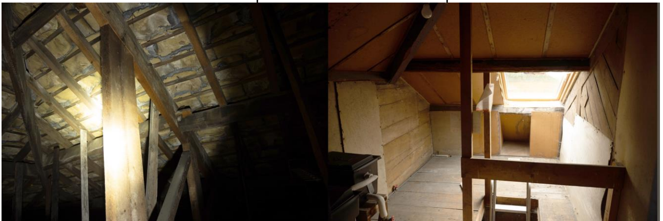
Photo 1: Illustrating roof interior.
