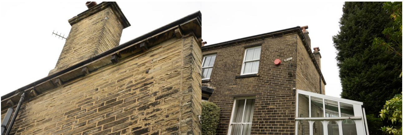
Photo 3: Showing flat stone gutter support and pointed walls
