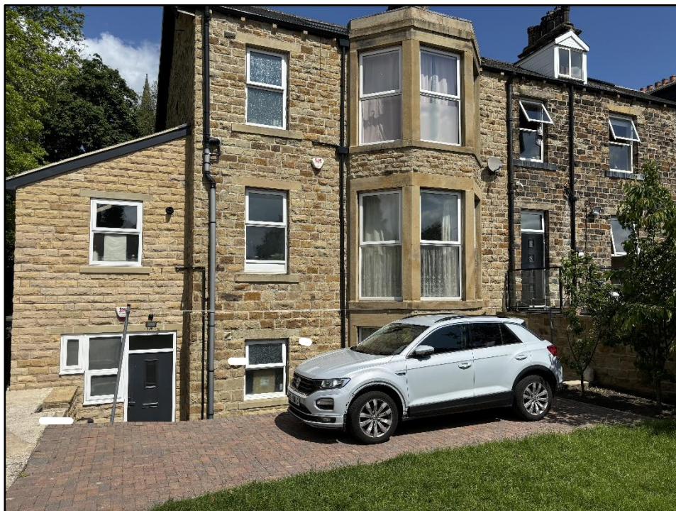
Plate 2: Rear elevation of site © 2024 Martin Walsh Architectural
