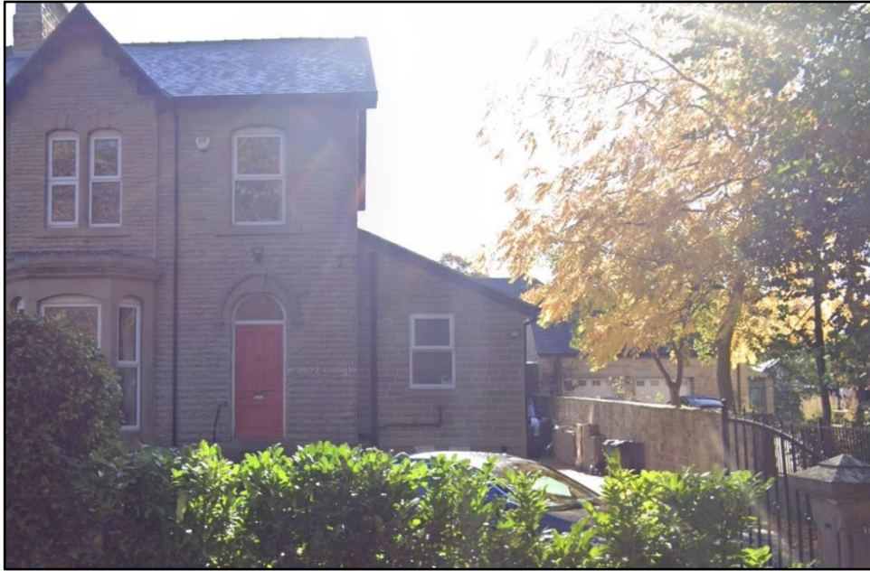
Plate 1: Front elevation of site © Google Streetview.
