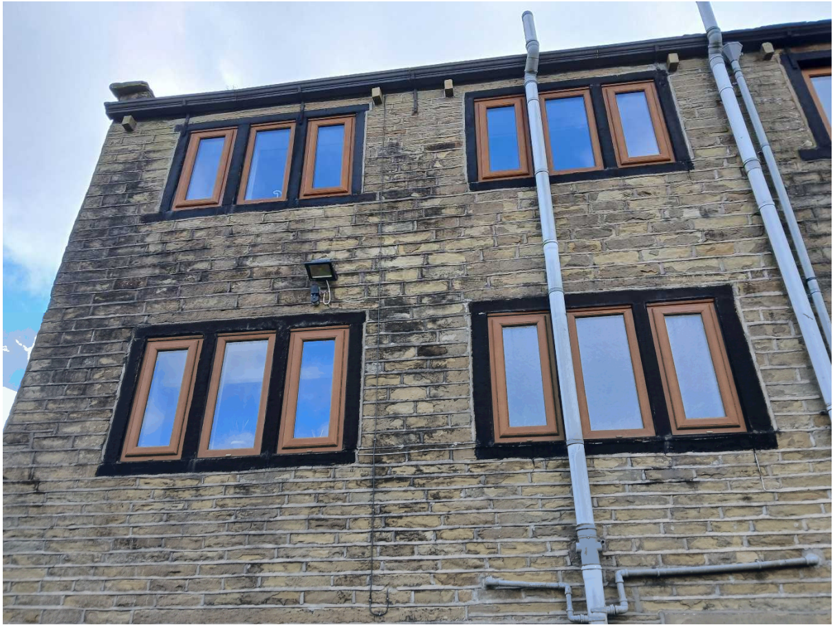
First and Second Floor Windows – 132 Gillroyd Lane
