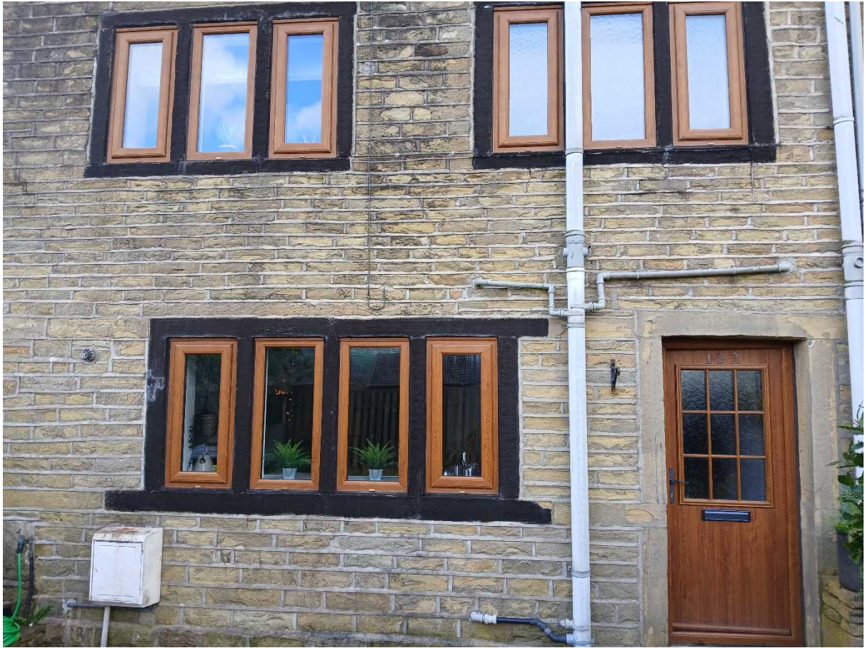
Ground and First Floor Windows and Door – 132 Gillroyd Lane
