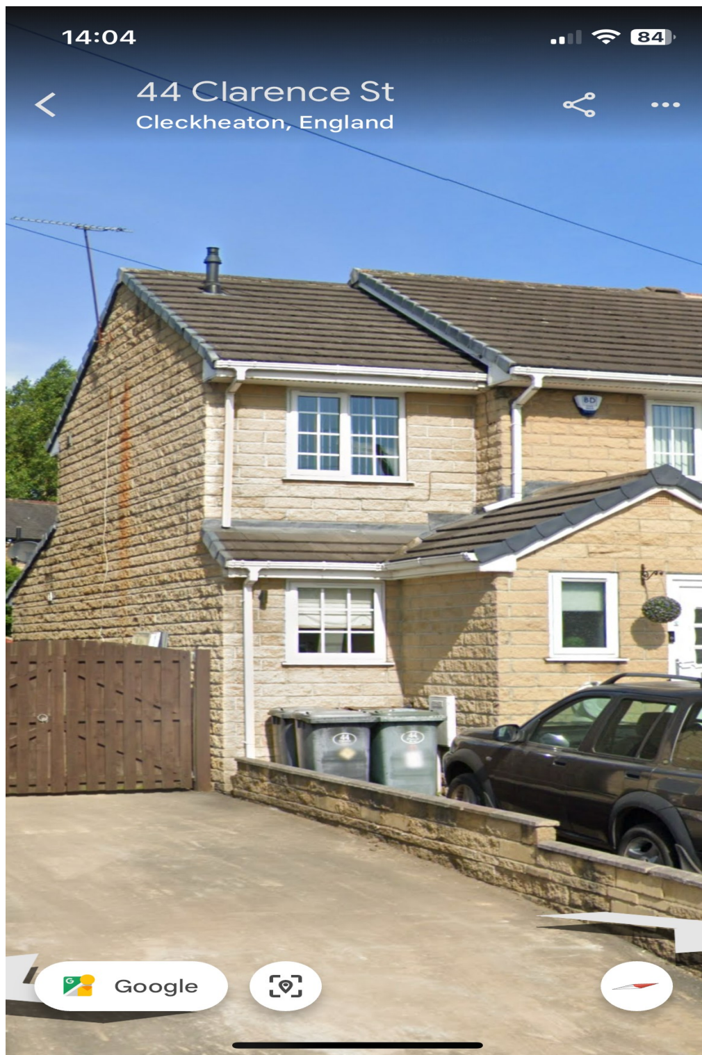
Full width side extension at no. 44
