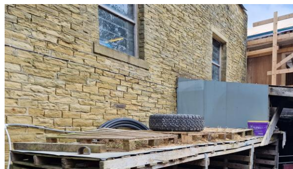
Rear elevation of the barn
