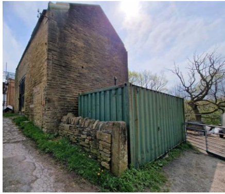
Storage container to the roadside elevation
