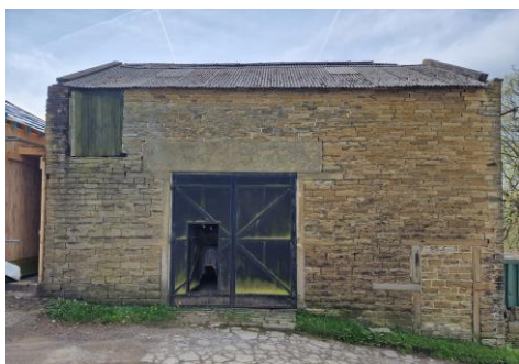
Front elevation of the barn
