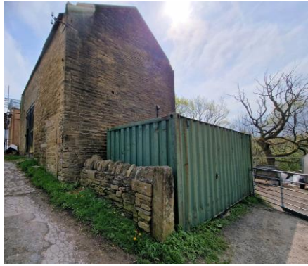
Storage container to the roadside elevation
