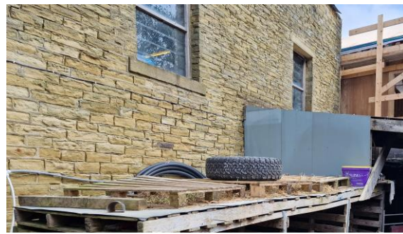
Rear elevation of the barn
