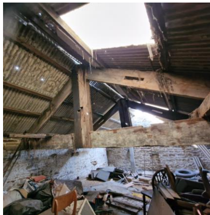
Upper floor and roof structure
