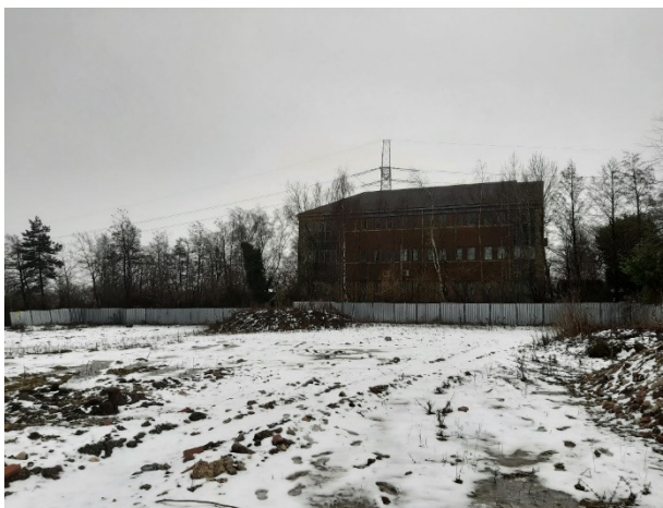
Photo 5: G23 at the southern boundary, screening the site from adjacent office buildings
