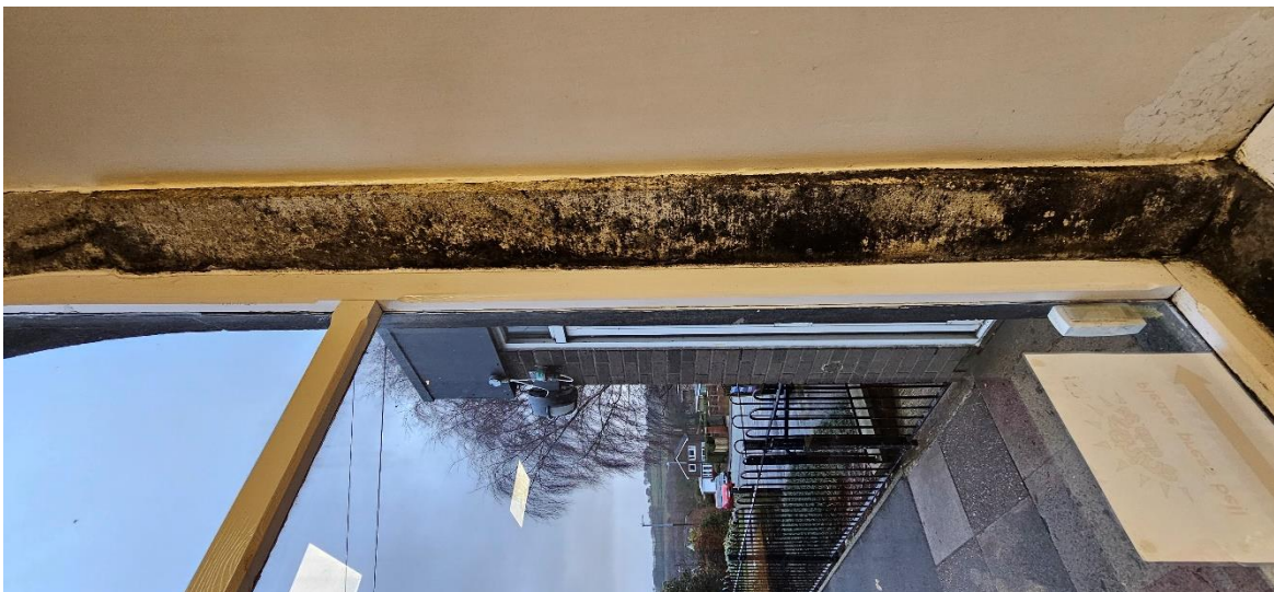
Photo 15: Uneven finish of stone and timber frame following contours of stone.
