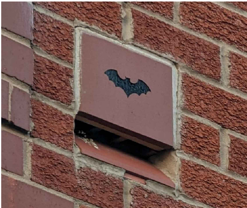
2no. Ibstock enclosed Type C bat box 215 x 215 x 105mm
