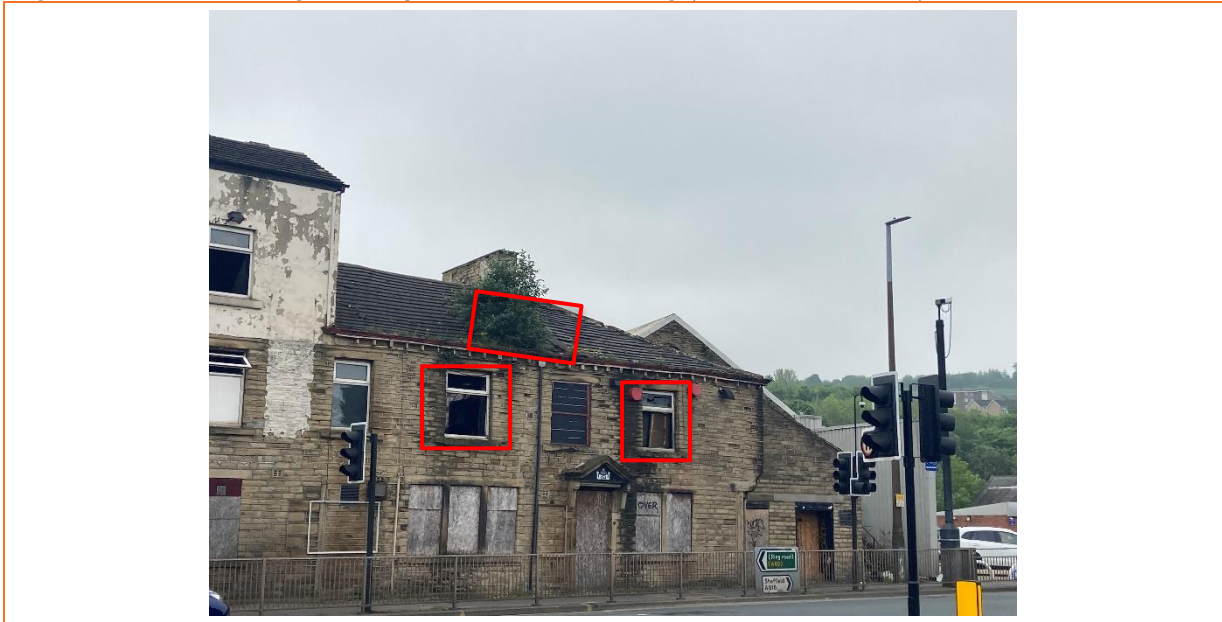
Figure 14 Showing access points into the building (AP4, AP5 and AP6)
