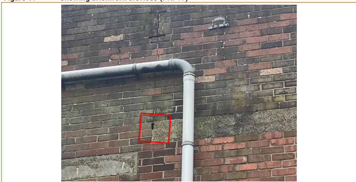
Figure 19 Showing brickwork crevices (PRF19)
