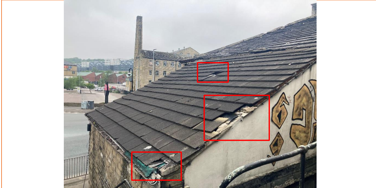
Figure 2 Showing the extension roof (PRF1, 2, 3)
