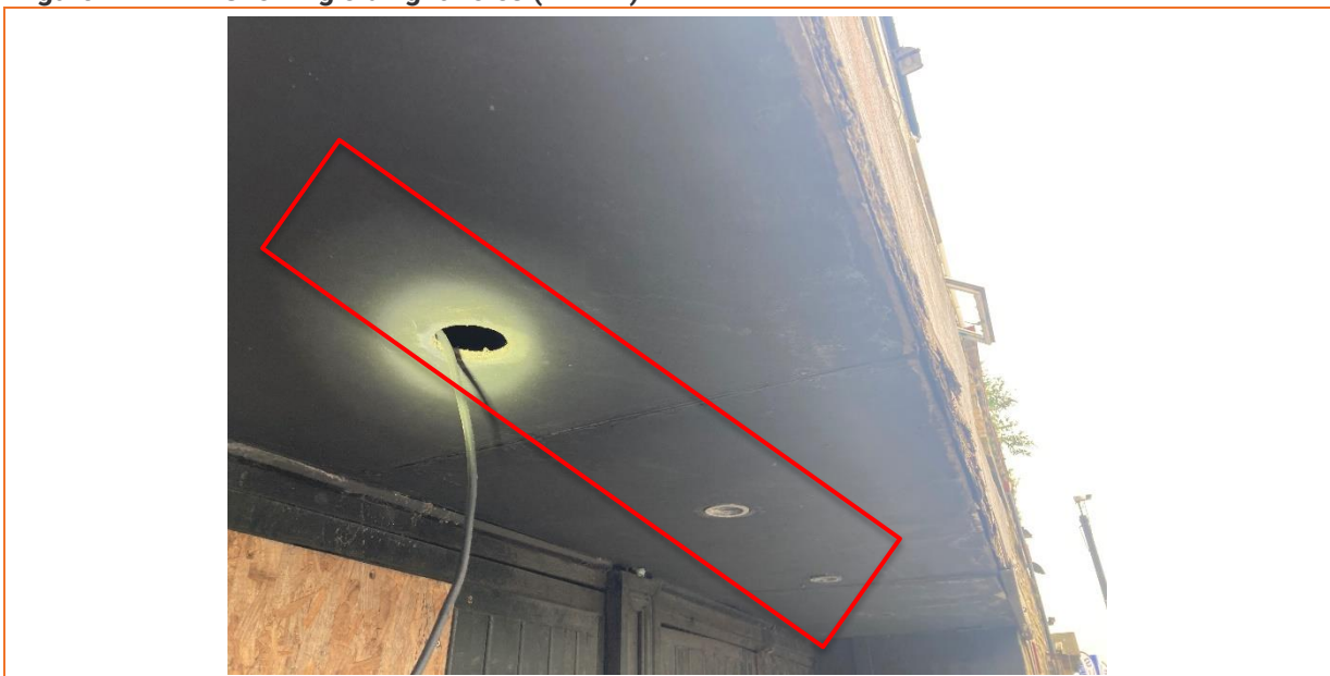
Figure 17 Showing old light holes (PRF17)
