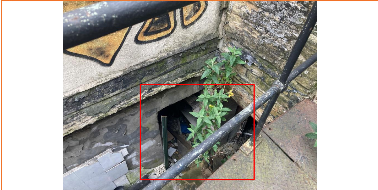
Figure 3 Showing an access point into the extension (AP1)
