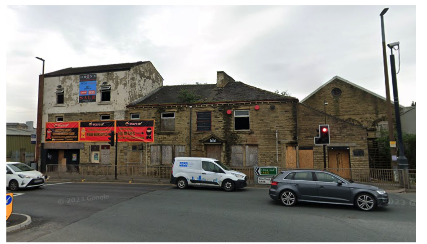
IMAGE SHOWING CONDITION OF BUILDING
