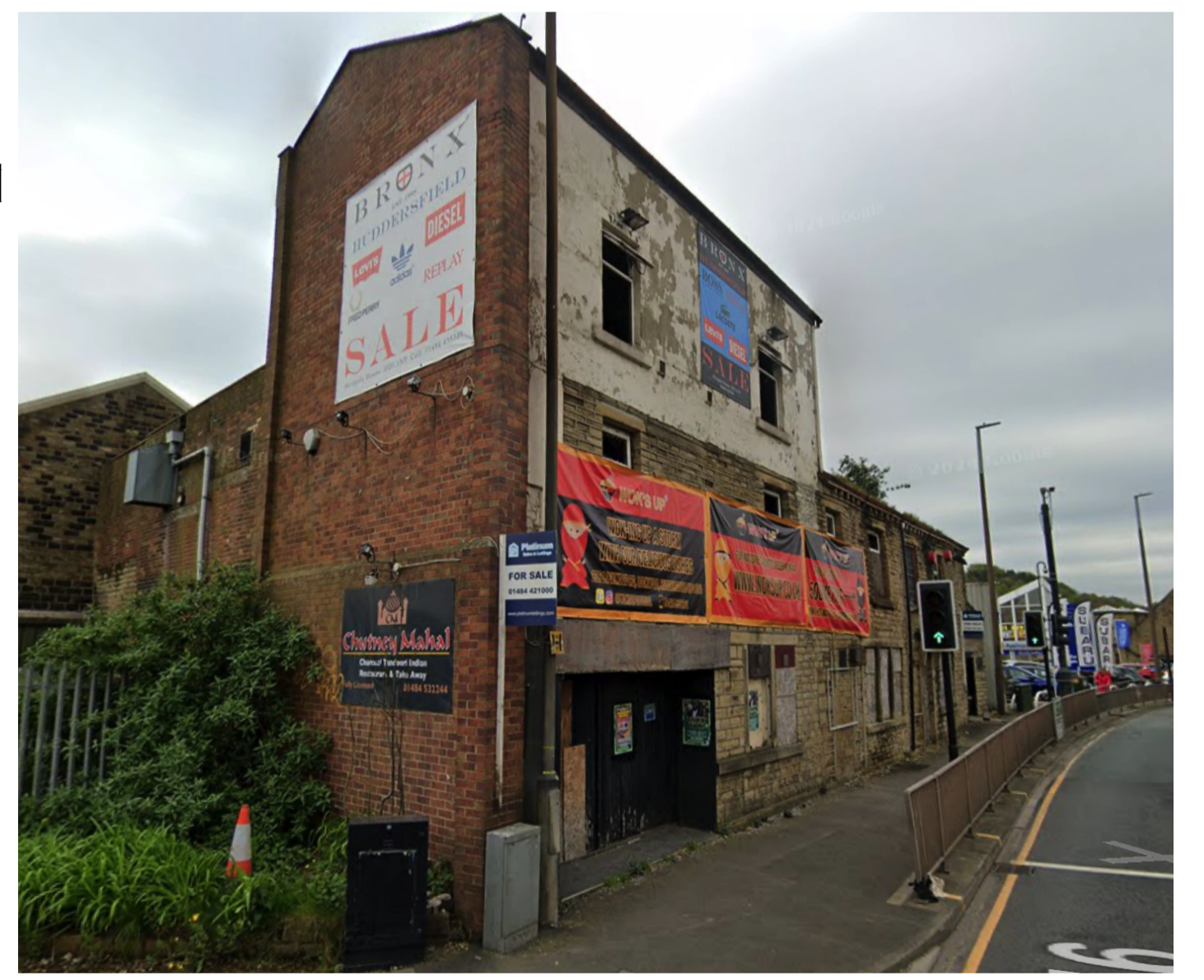
IMAGE SHOWING CONDITION OF BUILDING
