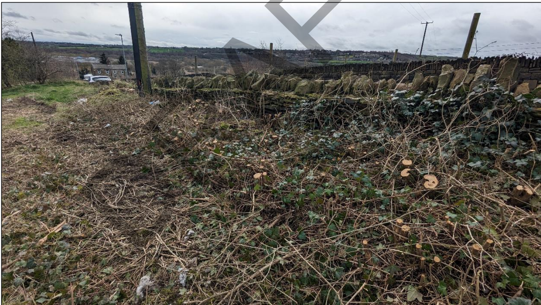
Photograph 2: Western boundary adjacent to Long Lane (subject to veg clearance)
