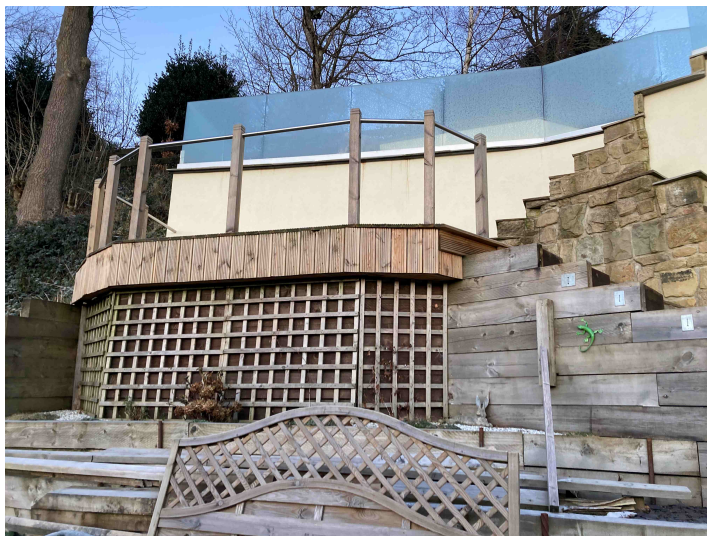
Photograph 1 - Existing Cream Coloured Rendered Garden Walls
