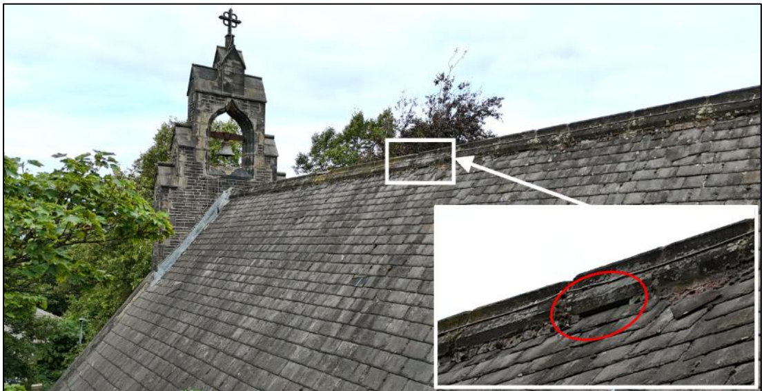
Plate 6. Gap behind flat-backed cast iron gutter
