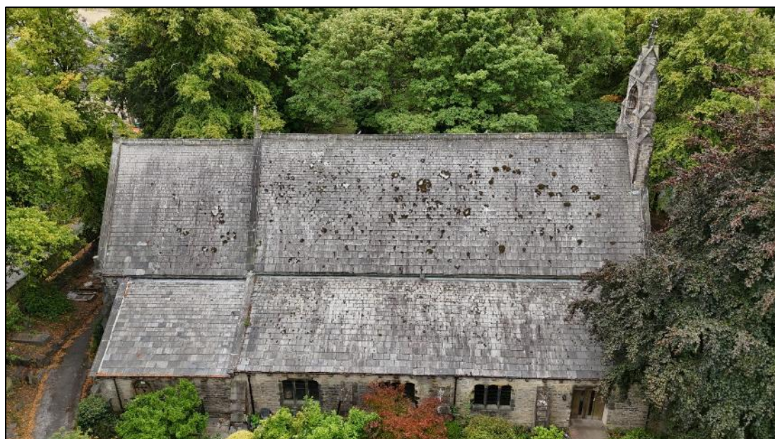
Plate 1. Northeast elevation of The Newsome Centre
