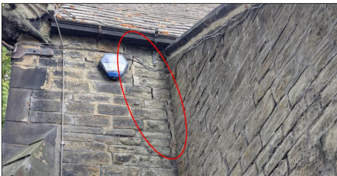
Plate 8. Crack in wall between southeast end of north aisle and northeast elevation of church
