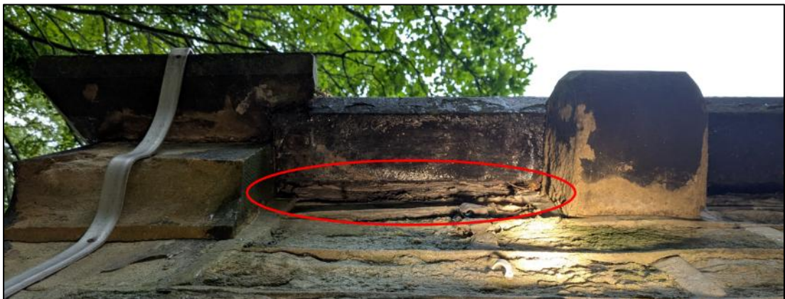
Plate 6. Gap behind flat-backed cast iron gutter
