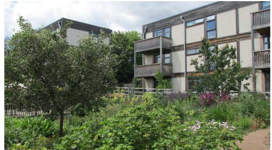
A car-free development comprising of energy efficient modular homes set around attractive SuDS infrastructure at LILAC, Leeds
