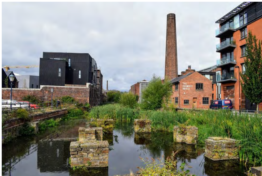
Combining industrial heritage and modern construction methods to create low carbon homes at Little Kelham, Sheffield (Image: Flickr/Academy of Urbanism)
