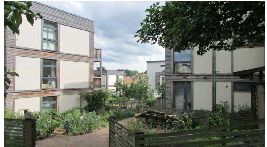
Buildings orientated for solar gain at LILAC, Leeds
