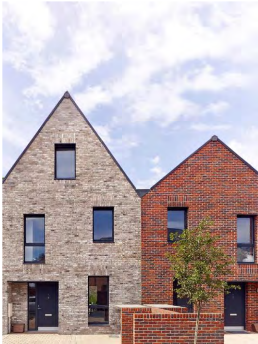
Contemporary window materials set back in deep reveals at St Chads Tilbury (Image: Kilian O'Sullivan www.kilianosullivan.com )
