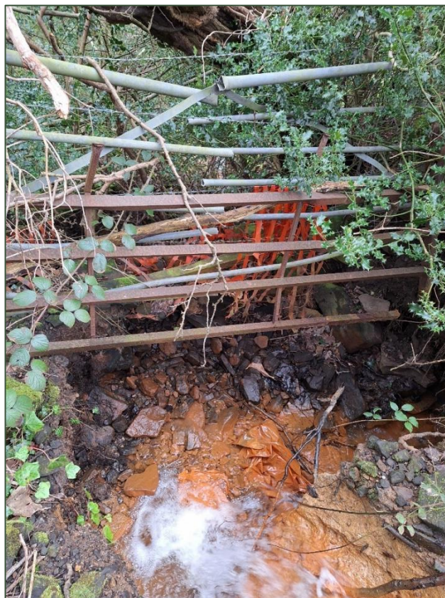
Plate 6 – Fencing material obstructing flows.
