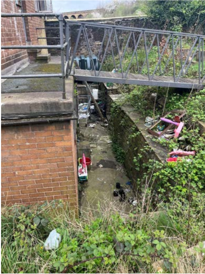
Figure 7 Rear of Building
