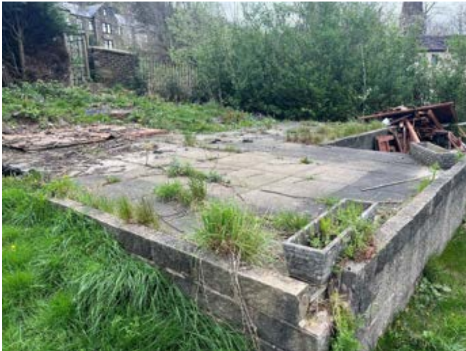
Figure 2 Foundation of former outbuilding
