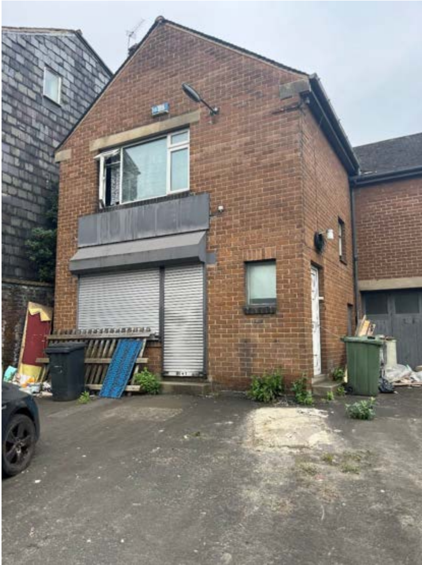
Figure 9 Front of Site off Manchester Road
