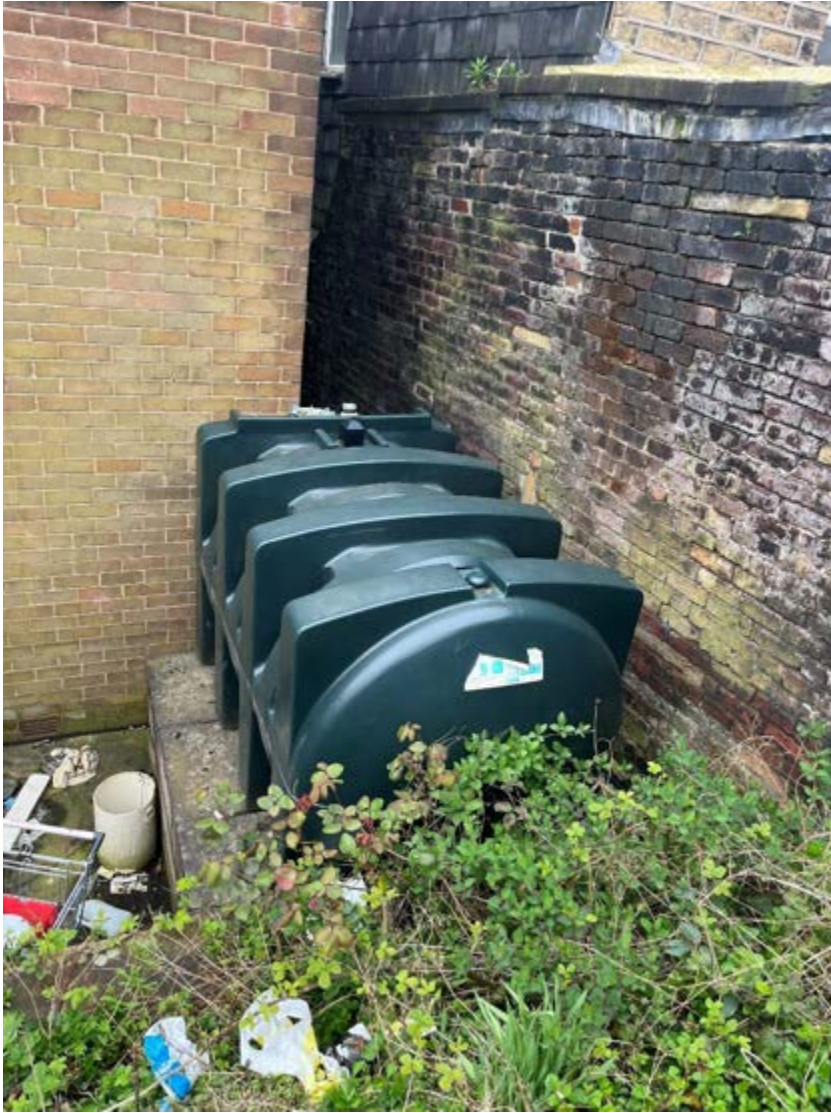
Figure 6 Storage Tank at rear of Building
