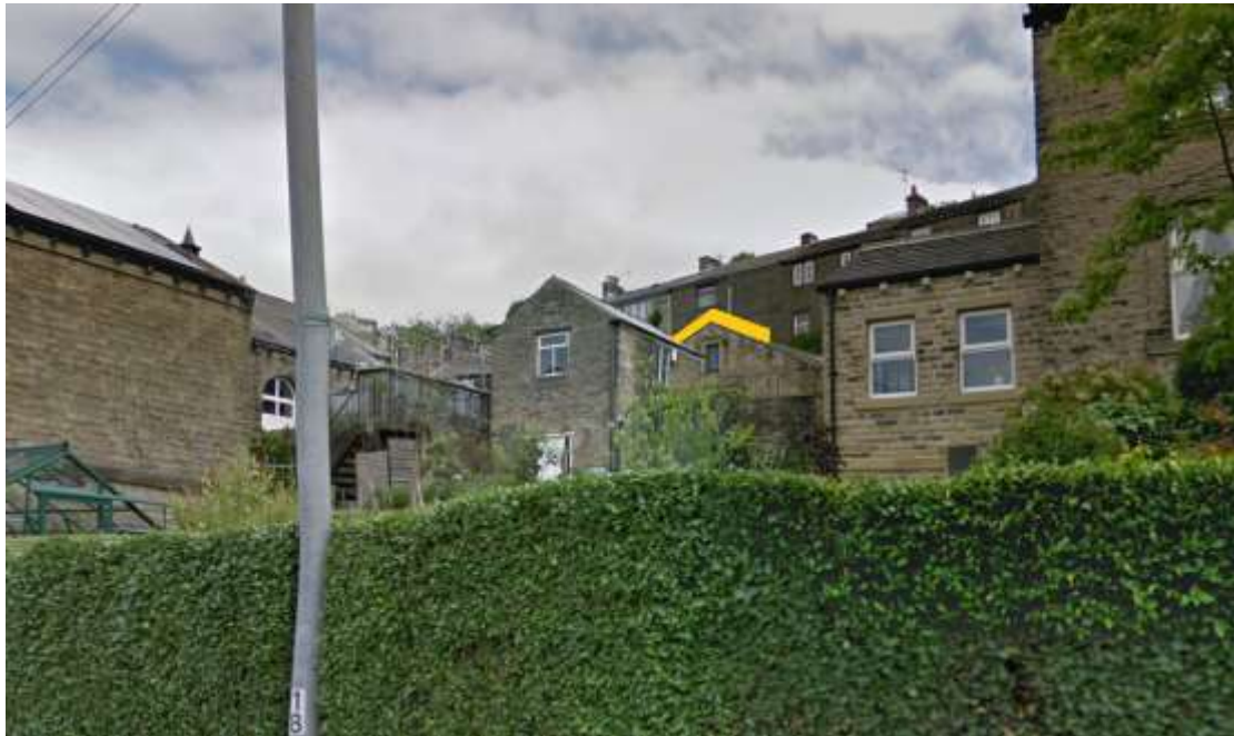
Annotated View from Dunford Road - Above
