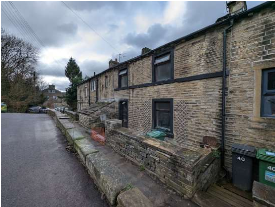
Underbank Old Road - Above
