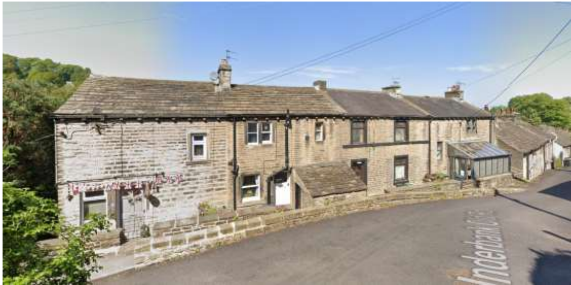
Underbank Old Road - Above
