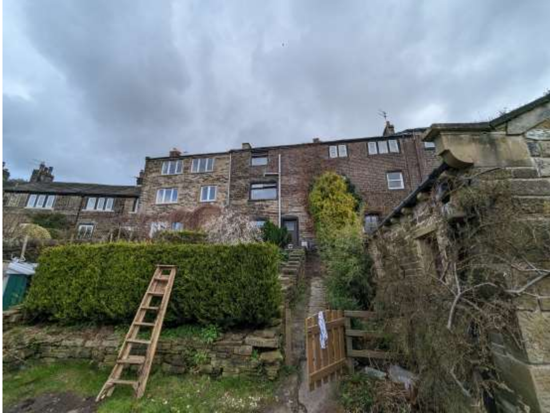
View from Low gate - Above
