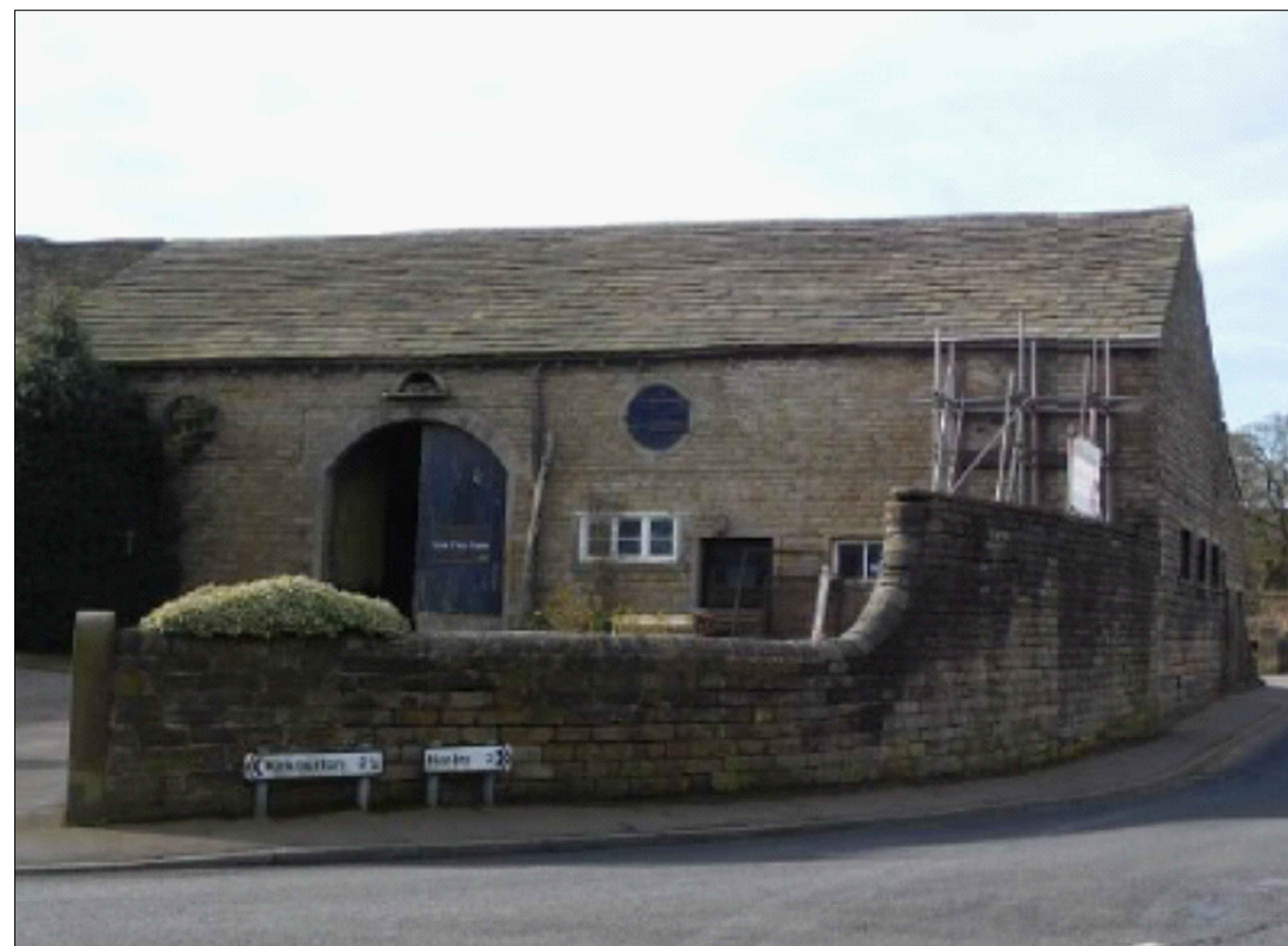
BOUNDARY RETAINING WALL - AS EXISTING
