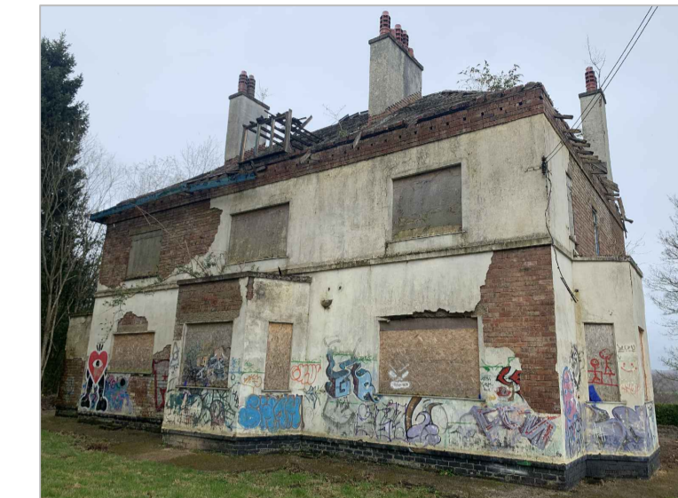
Rear Elevaton (SW Facing)
