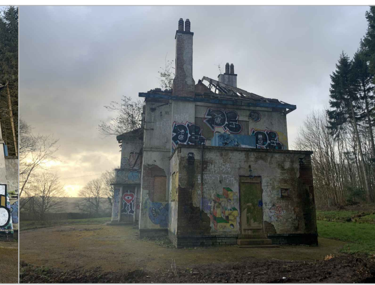
Side Elevaton (NW Facing)
