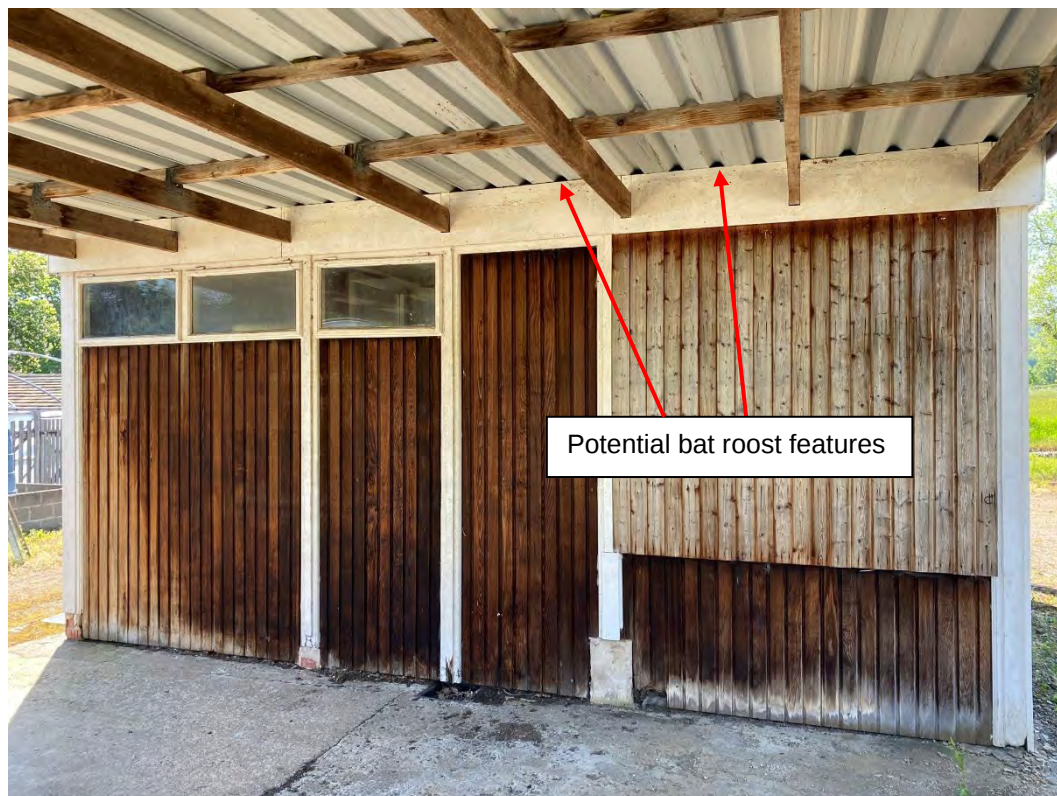
Photo 6. North elevation of building on the site
