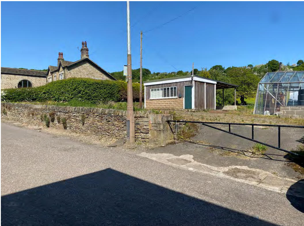
Photo 2. Looking north-west towards the south-western part of the site
