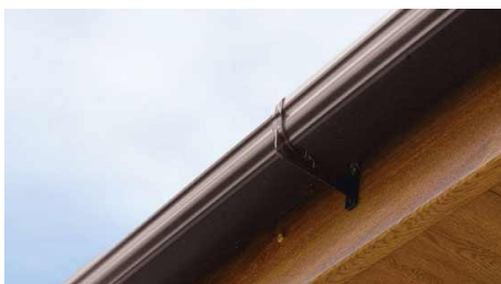
Brown plastic rainwater goods on oak effect uPVC fascias
