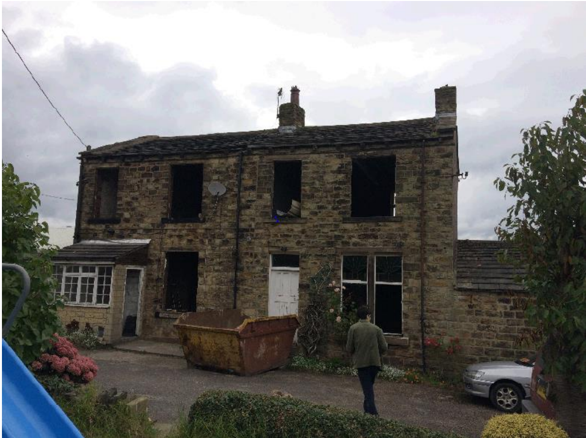
Image 1 - Separate House with Porch to be Demolished
