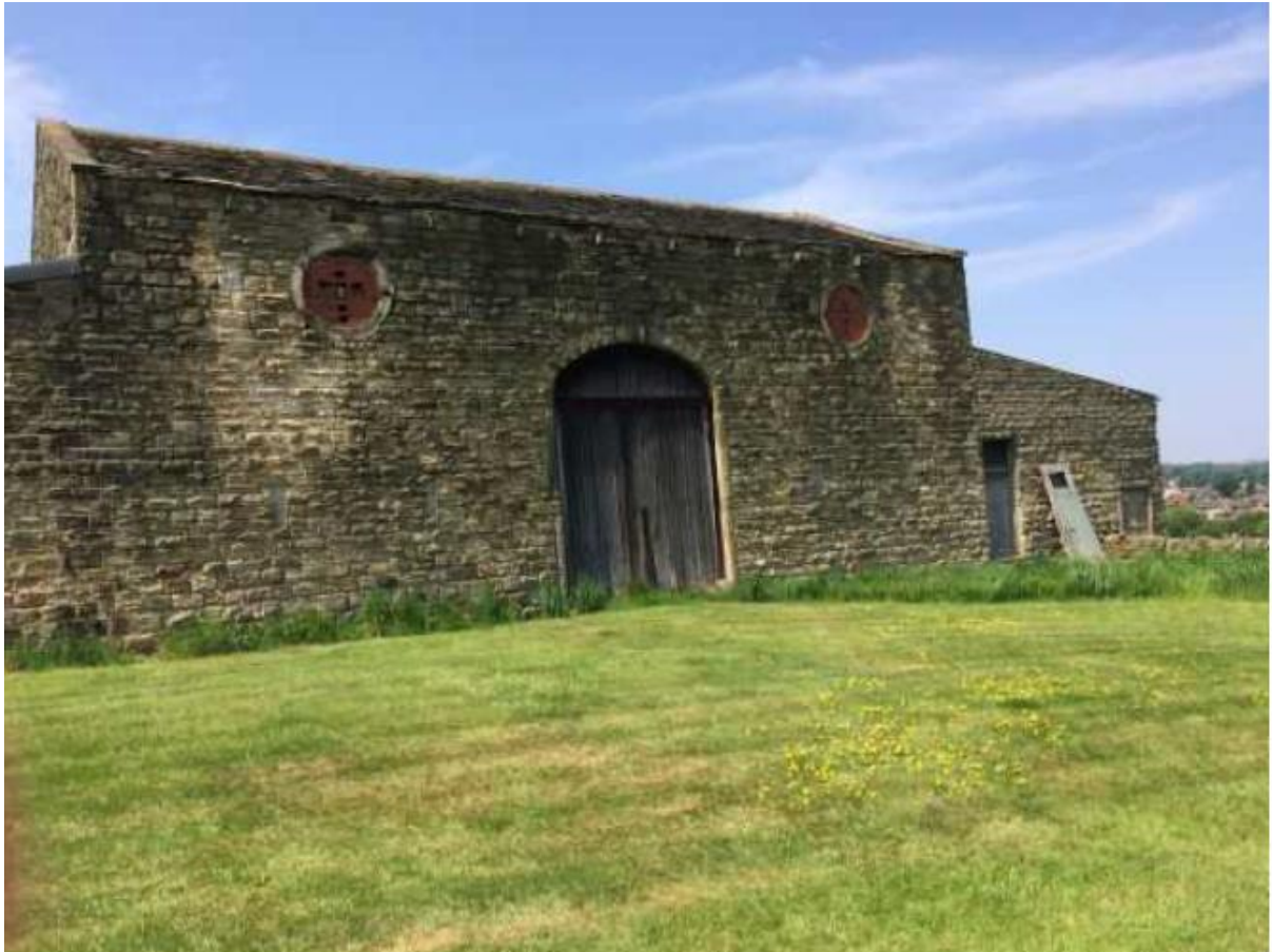
Image 5 - Front Elevation of Stone Barn
