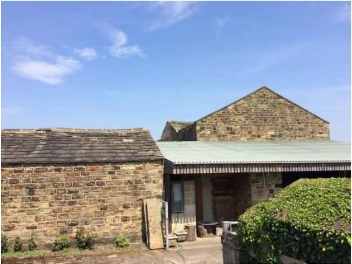
Image 4 - End of Garage and Relationship to Farm Outbuildings
