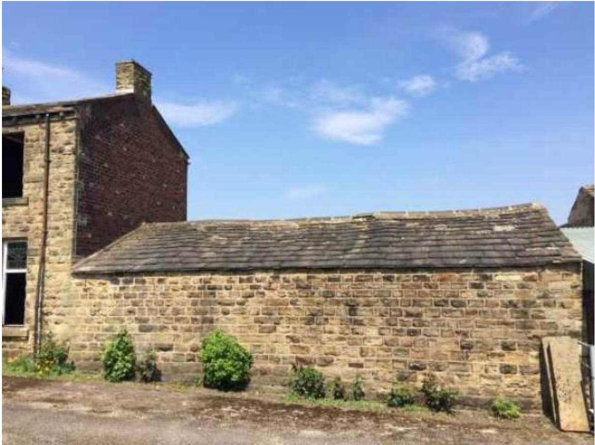
Image 3 - Existing Garage Building (to be raised)
