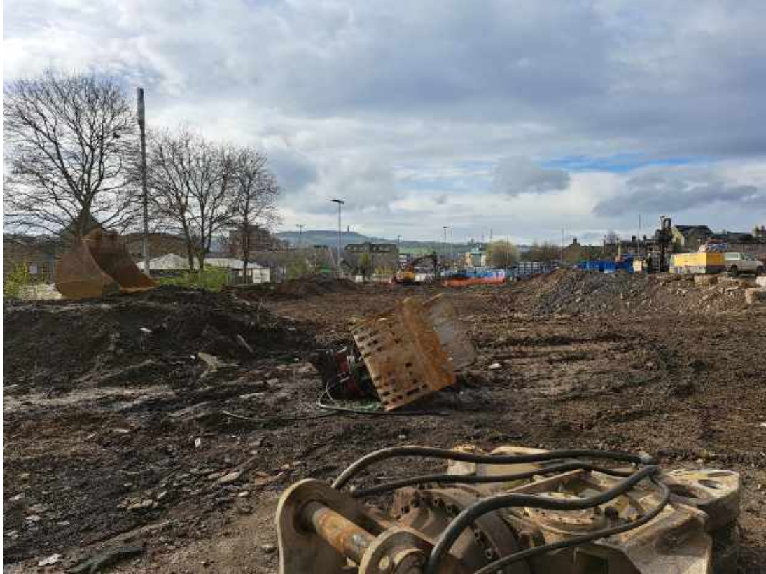
Photograph 3 View south from northern boundary.
