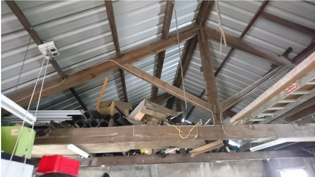
Figure 4: Internal view of the roof in the Workshop.
