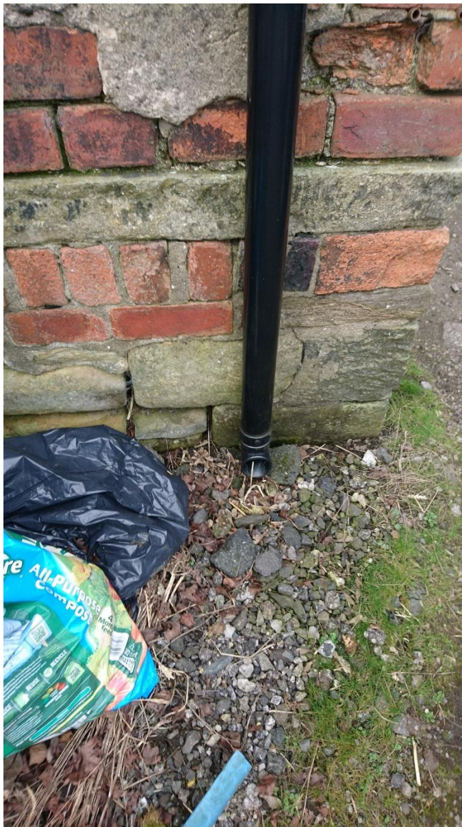
Figure 14: Detail view of the drainage provision to the downpipe on the eastern corner.
