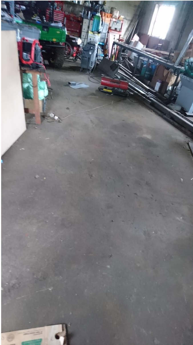
Figure 15: The smooth concrete floor provision.
