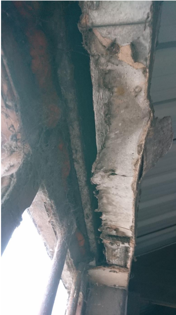
Figure 9: Internal timber lintels and cavity in the north-western elevation
