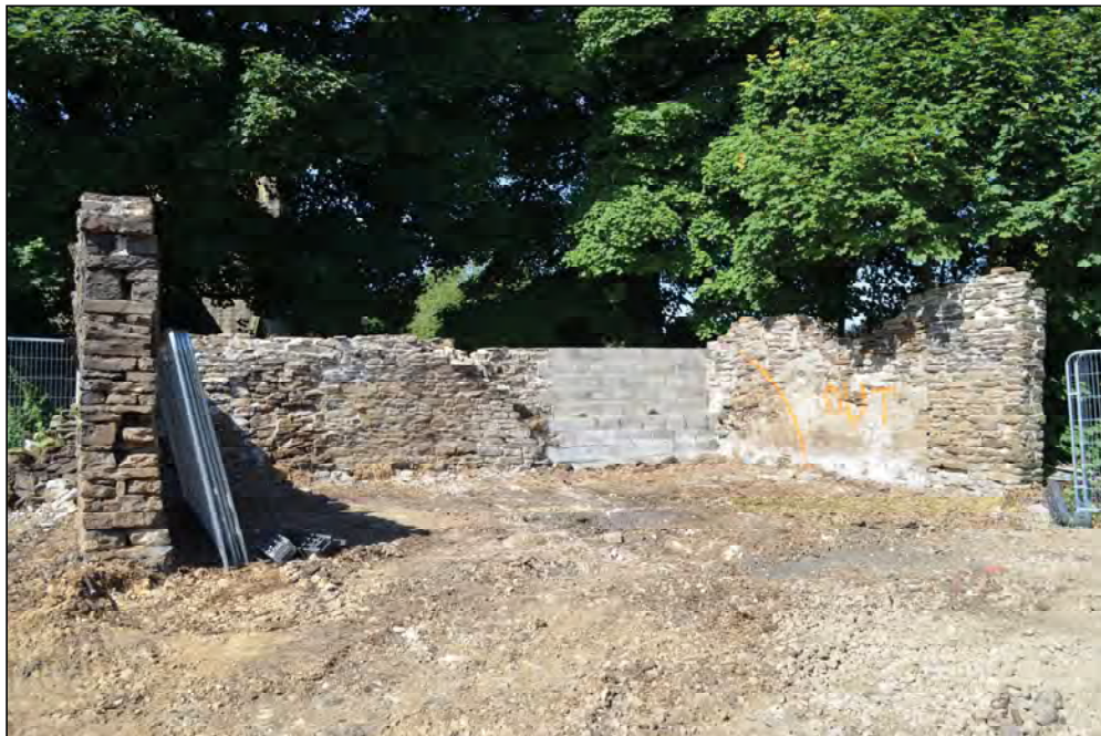
Plate 20. Structure 7, prior to demolition, looking west
