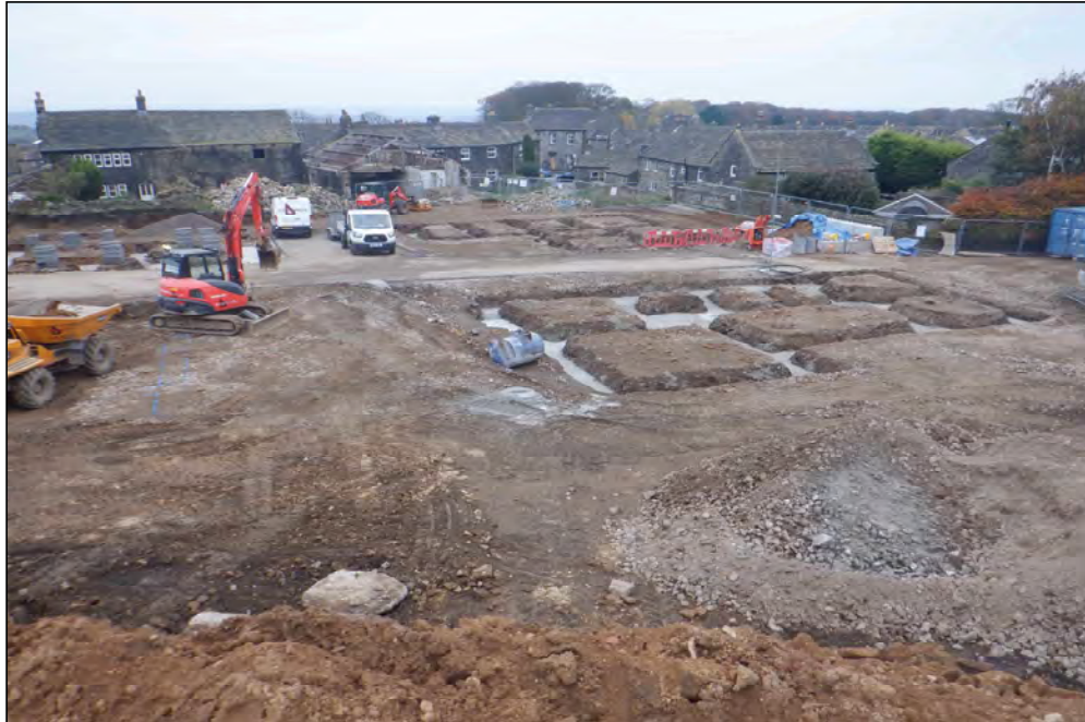
Plate 9. Foundation trenches at the eastern edge of the site, looking north
