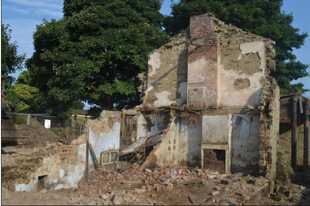
Plate 5. Partial demolition of Structure 5
