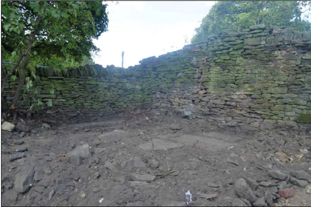
Plate 23. Structure 10, looking northwest
