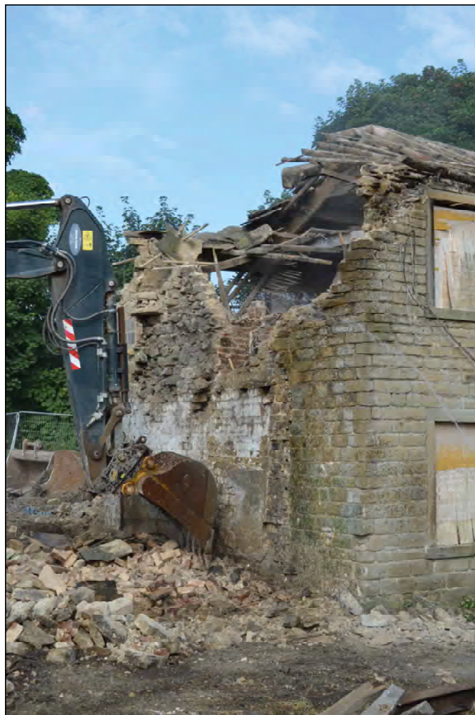
Plate 4. Demolition of the southern elevation of Structure 5, looking west
