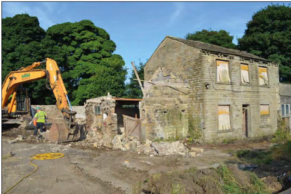
Plate 2. Demolition of Structure 5, looking west
