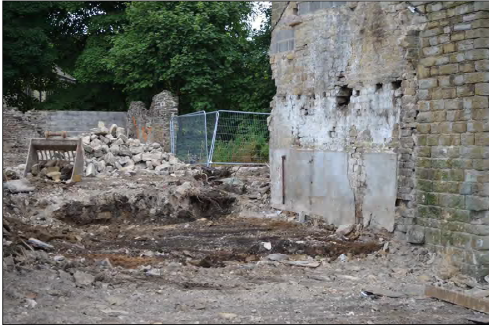
Plate 3. Structure 5 following demolition, looking west
