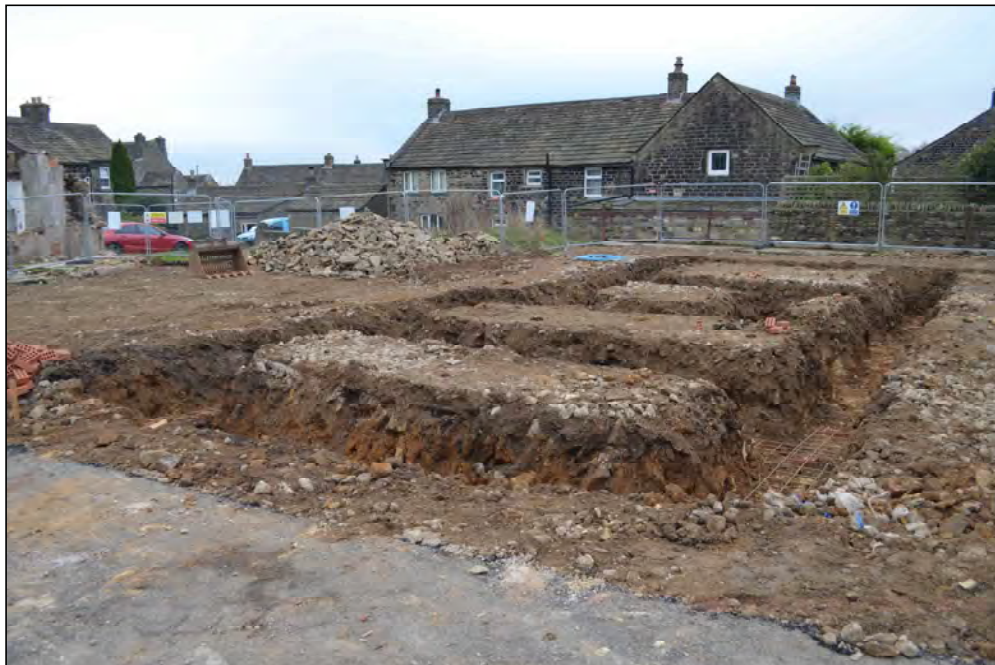
Plate 8. Foundation trench at the eastern edge of the site, looking northwest
