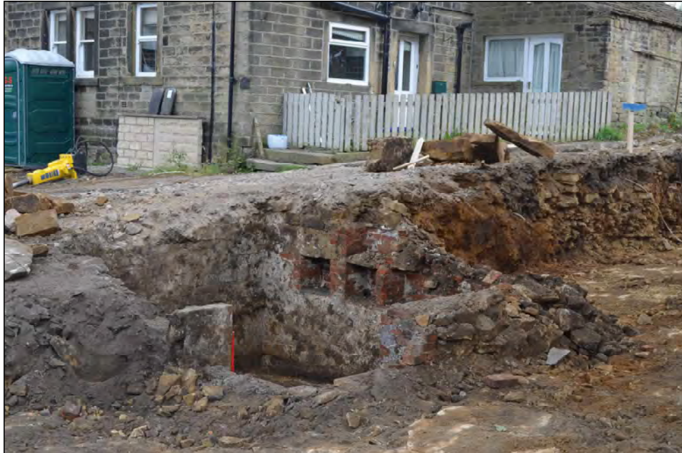
Plate 17. Structure 6, cellar, looking southeast
