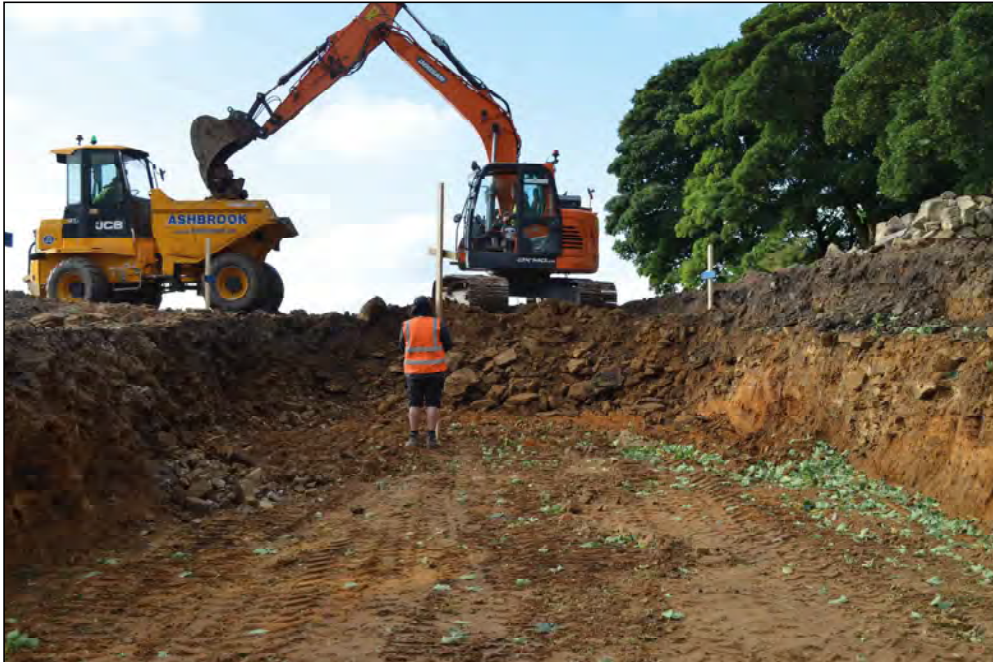
Plate 6. Excavation of the new roadway into the site, looking south
