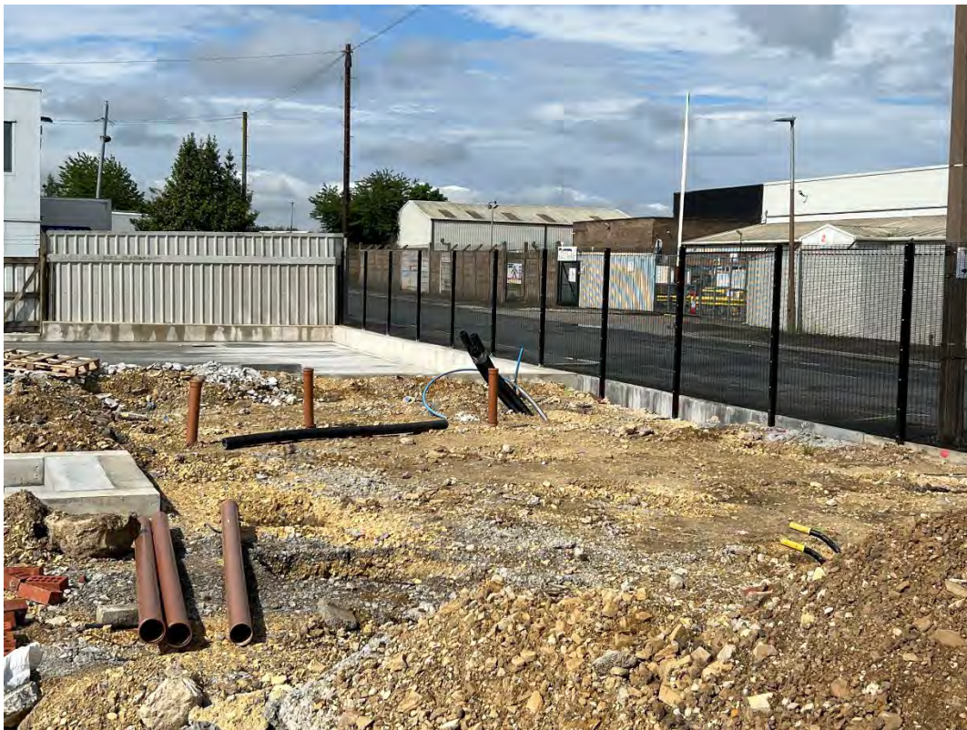
Photograph No.4: Northern boundary facing west.
