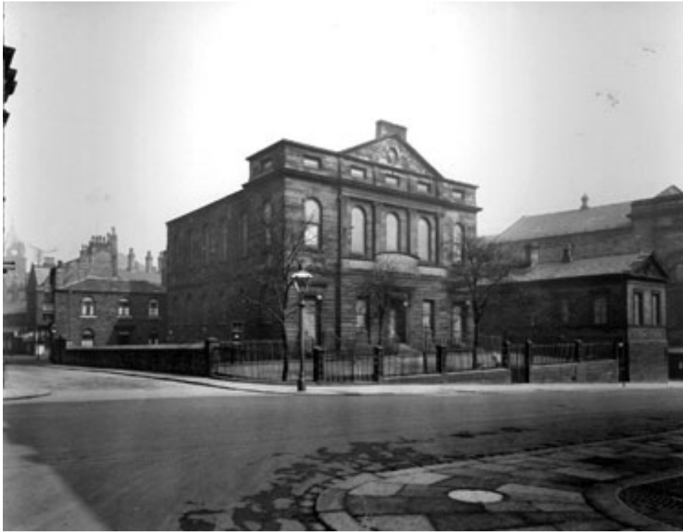
Plate 24 View of Ramsden Street Congregational Church viewed from corner of Victoria Lane and Ramsden Street – note level change on western elevation (stairs down just out of shot) also not lack of room for burials externally.
