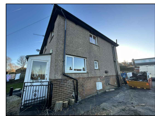
EXISTING PHOTOGRAPH - SIDE
