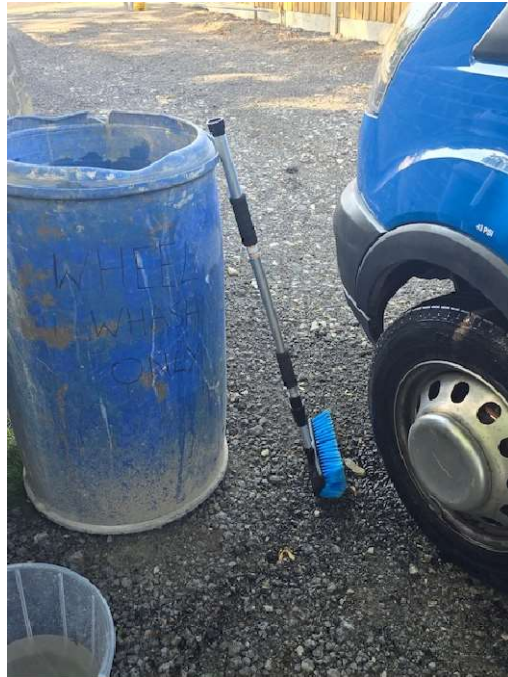
Photo's of wheel washing facilities at site entrance / exit.
