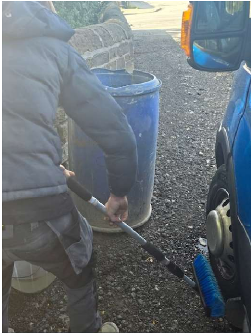
Photo's of wheel washing facilities at site entrance / exit.
