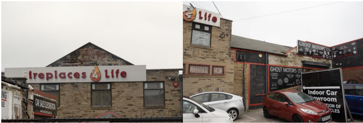
Photo 1: Showing gable and roof of building 1
