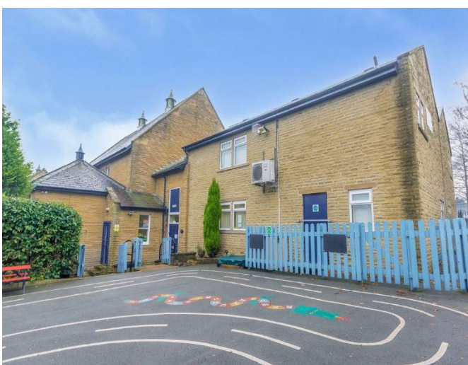
Figure 5 (above) – The existing paling fence to be repainted.
