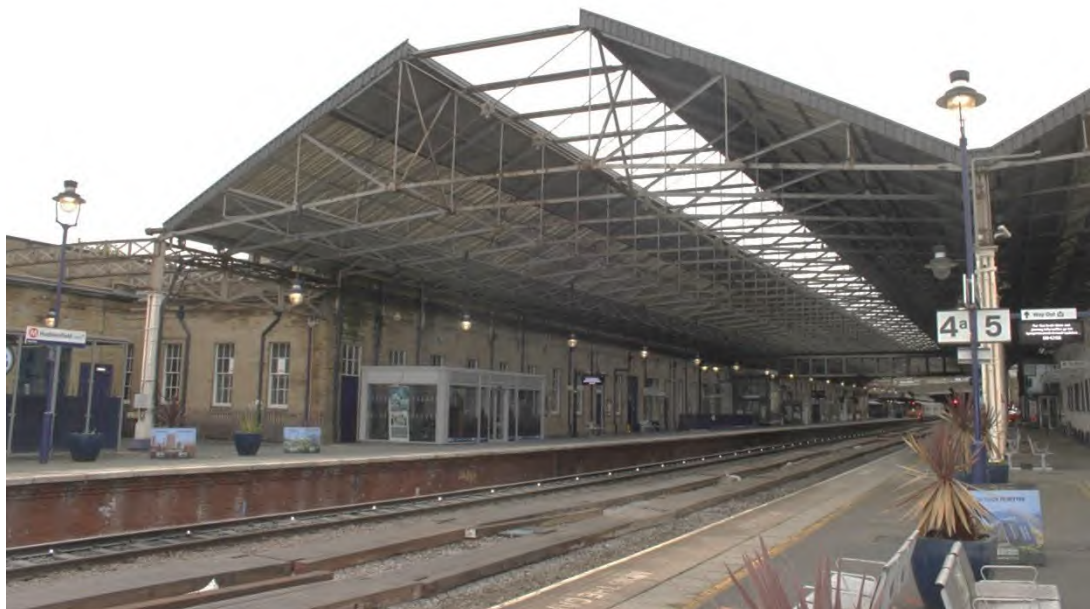
Plate 11: Northern gable end of Roof A, facing south-east
