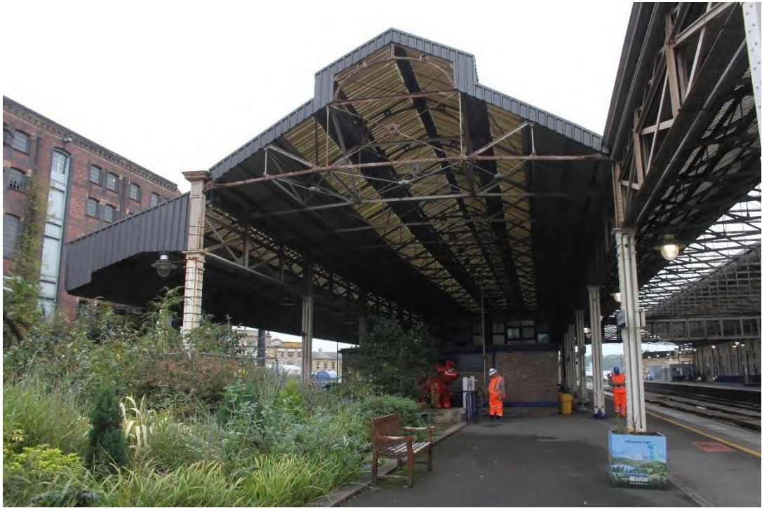
Plate 55: Southern elevation of Roof B with Roof A attached (right), cantilevered Roof C attached (left) and Large Brick Warehouse (1228533), facing north
