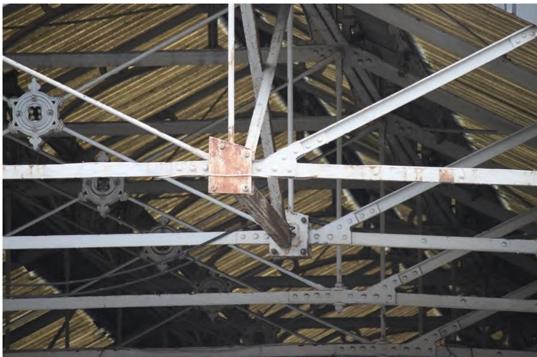
Plate 47: A later supporting bracket located at the western corner of the central cross brace
