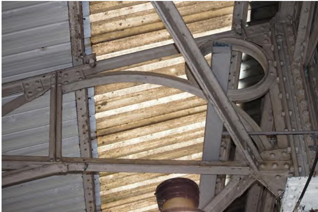
Plate 73: Example of eastern end of a riveted lattice wrought iron bracket attached to the western composite lattice beam of Roof B (right)
