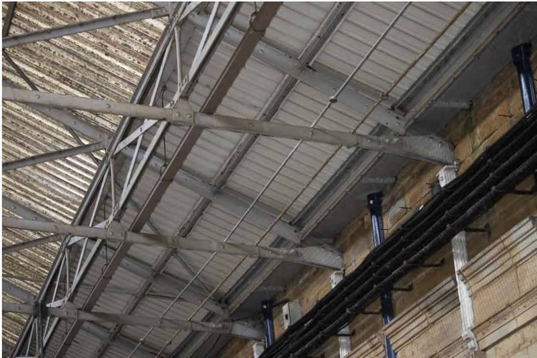
Plate 30: Structural supports with trusses attached above
