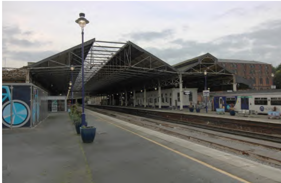
Plate 10: Northern gable end of Roof A (left) with attached Roof B (right), Roof C cantilevered off the edge of Roof B (far right) and the Large Brick Warehouse NHLE 1228533 (background far right), facing south-west
