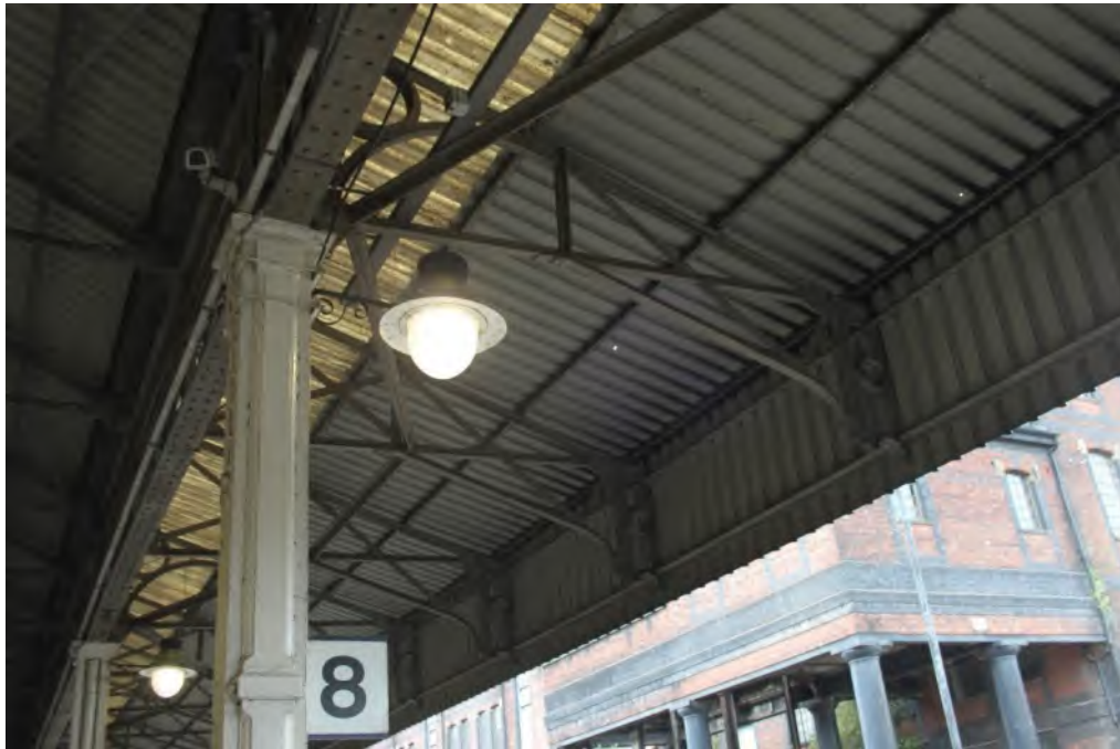
Plate 71: Example of riveted lattice wrought iron brackets within Roof C With the Large Brick Warehouse (NHLE1228533) (background left), facing south-west
