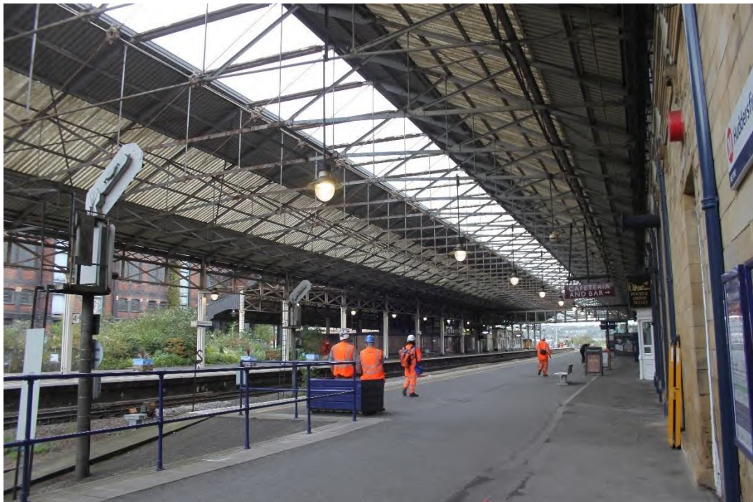
Plate 41: View of underside of Roof A, facing north
