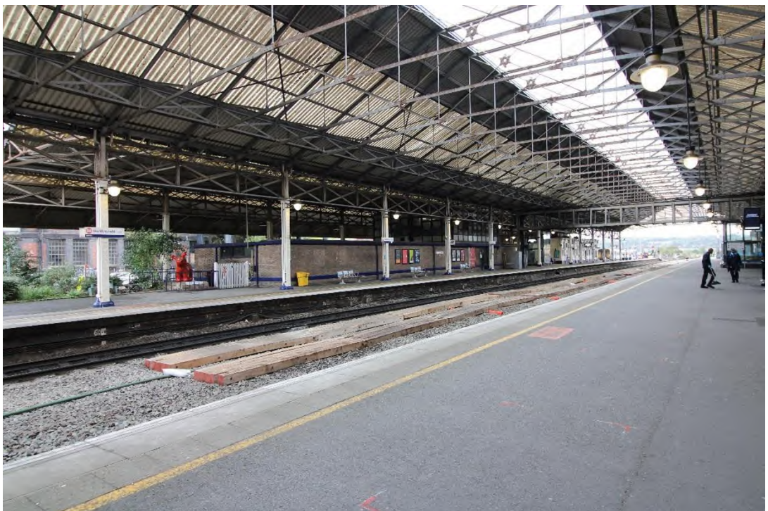
Plate 34: Central section of western elevation facing north-west
