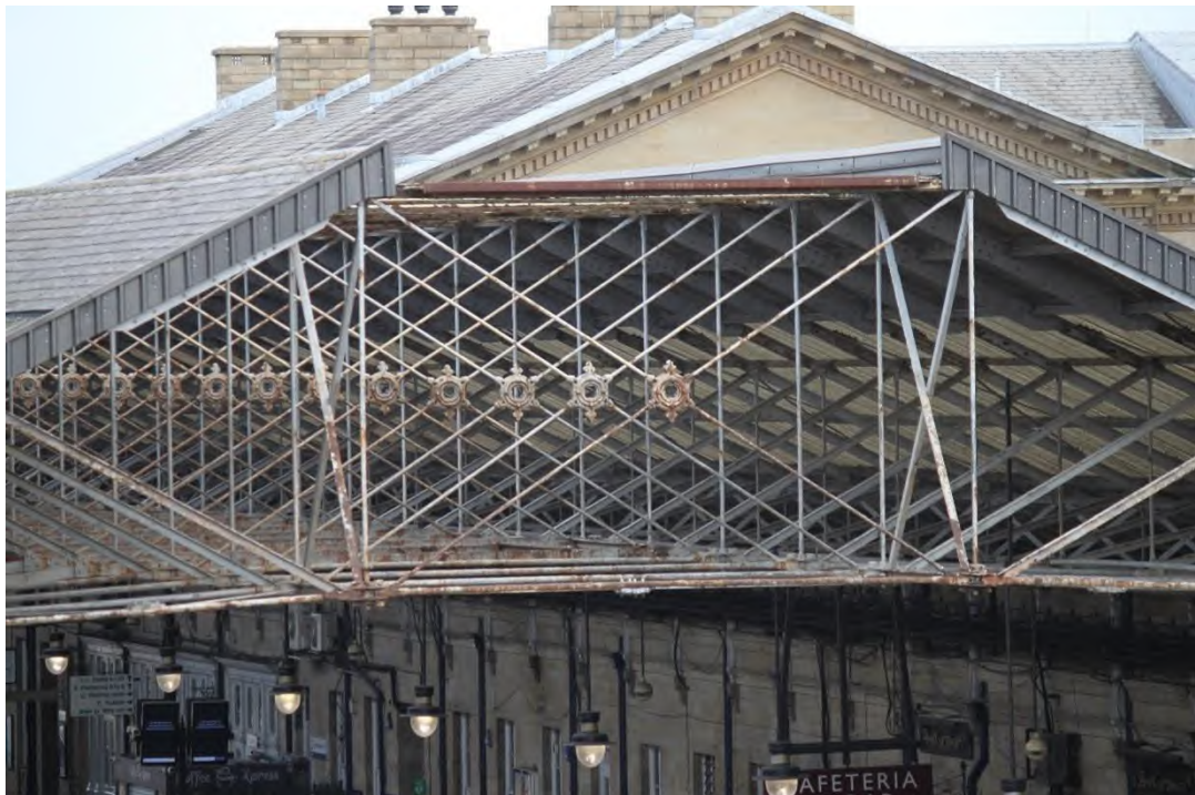
Plate 22: Central cross brace with elaborate central moulded roundel with the space above marking the location of the former roof lantern, facing north-east
