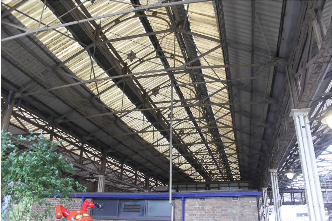
Plate 64: Underside of Roof B and lantern, north-west
