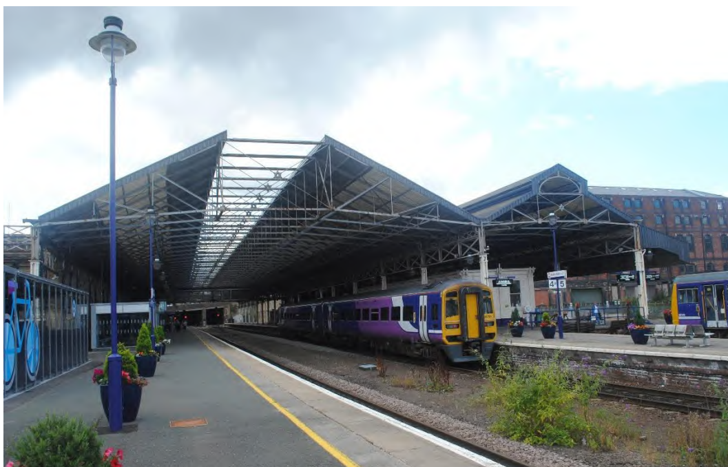
Insert 4-5 Trainshed roofs viewed from the northern end of the platforms, showing gable ends of principal ‘Roof A’ (left) and ‘Roof B’ (right). ‘Roof C’ is visible cantilevered off the edge of ‘Roof B’ on the far right.
