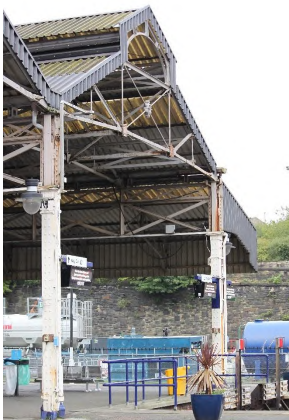
Plate 48: Northern gable end of Roof B with wrought iron column supports, facing west
