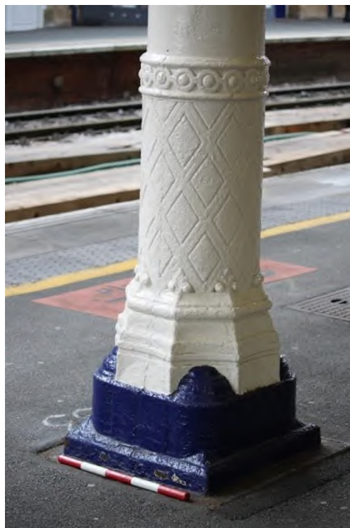
Plate 40: Decorative base of cast iron column with 0.5m scale
