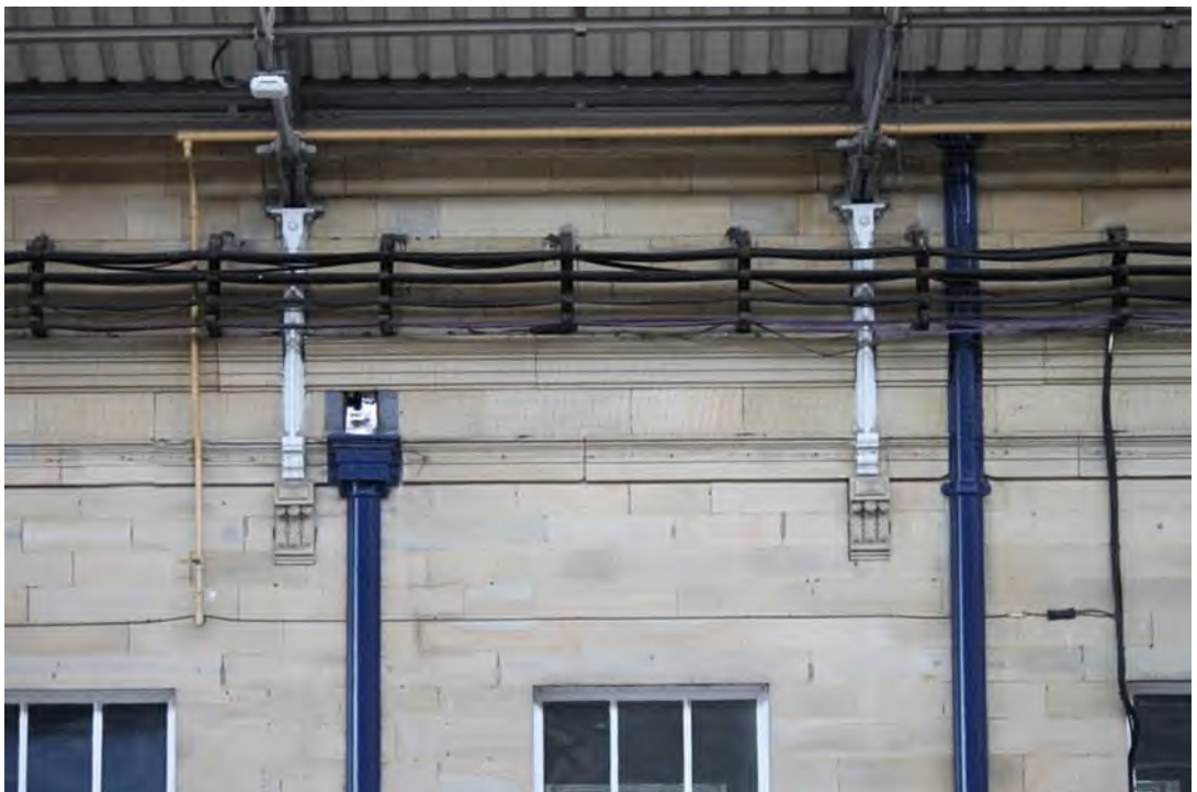
Plate 31: Example of two structural supports attached to the eastern elevation
