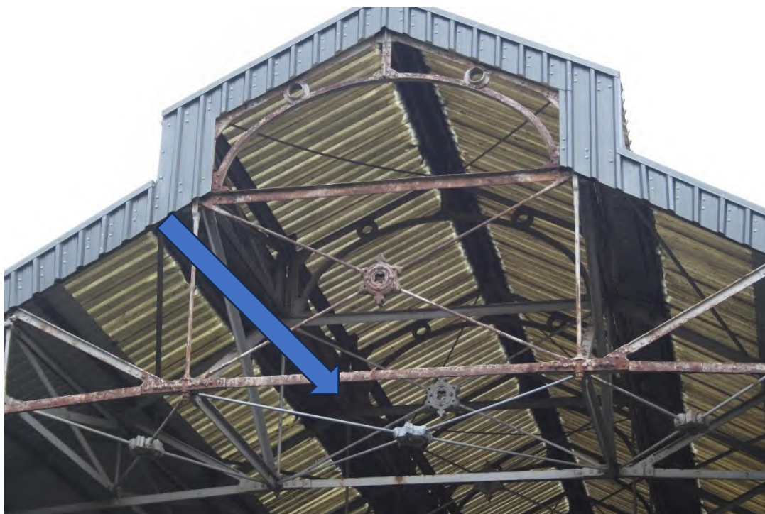
Plate 66: Decorative moulded fleur-de-lis roundels (bottom) laid perpendicular to the upright central cross bracing members at the southern end of Roof B, marked by arrow
