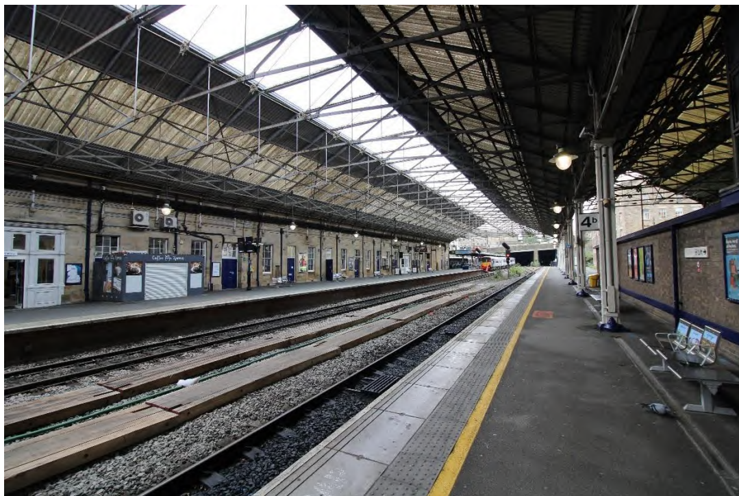
Plate 29: Southern end of eastern elevation (western elevation of station), facing south-east)
