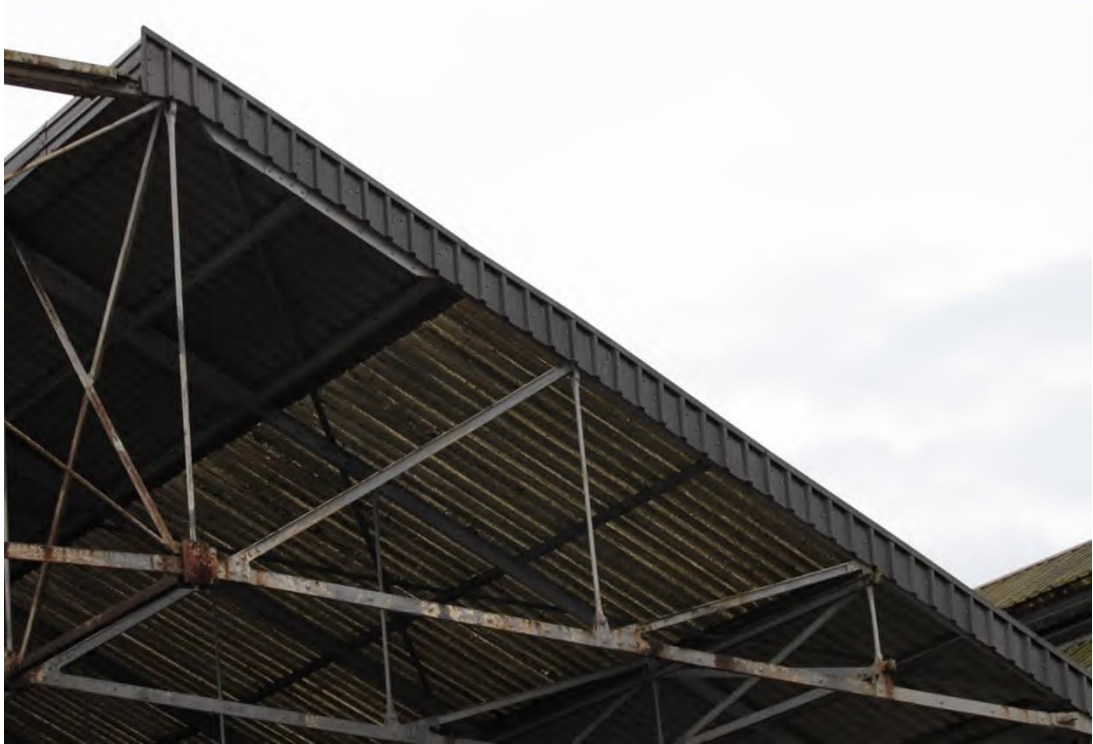
Plate 12: Western end of Roof A showing joist, struts and tie rod interlocked with joint plates and rivets
