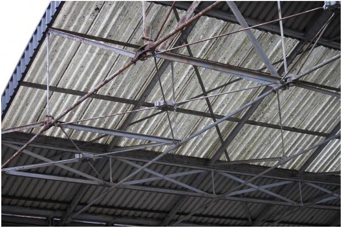
Plate 42: Manchester end of Roof A with tubular rafter ties and decorative moulded fleur-de-lis roundels laid perpendicular to the upright central cross braces
