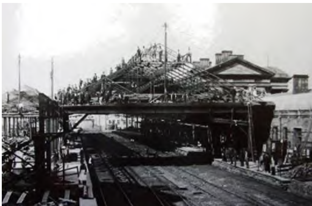
Plate 2: Trainshed roofs under construction, 1886 (Network Rail 2021)
