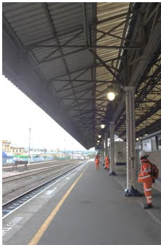
Plate 51: Lower western elevation of Roof B, facing north
