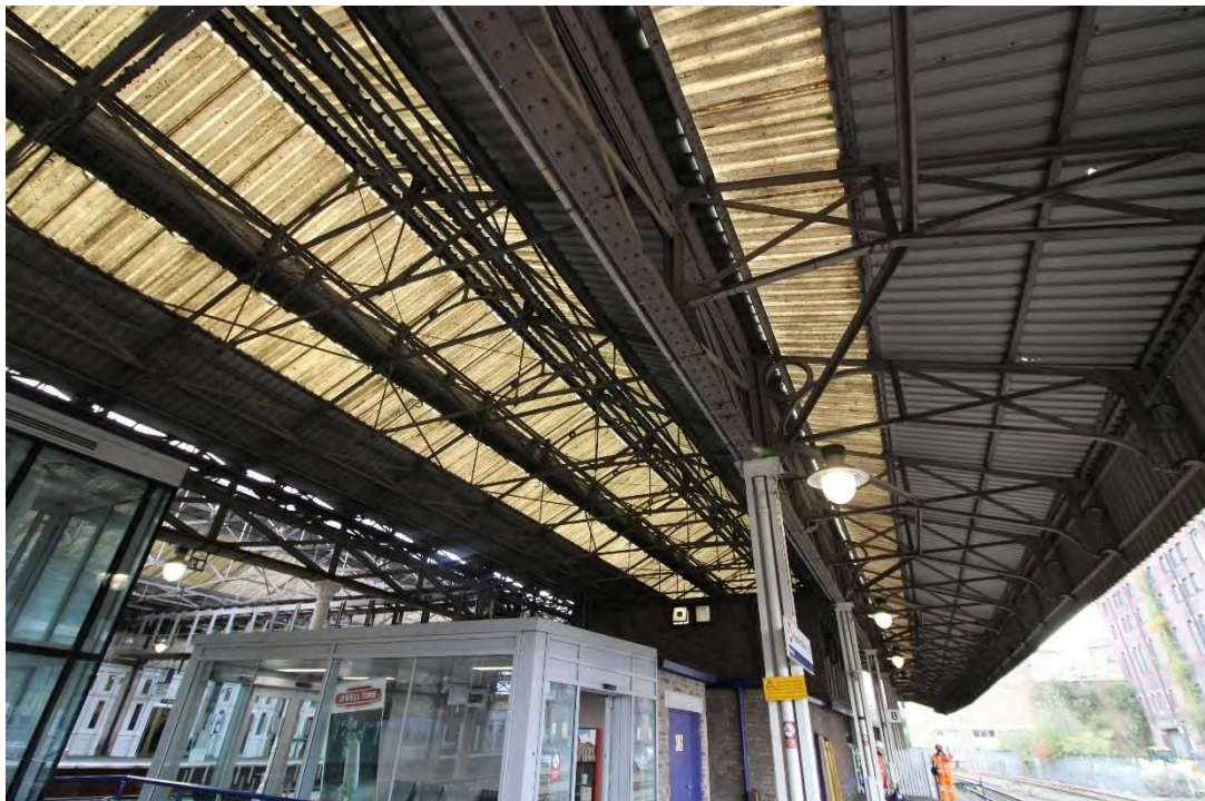
Plate 53: Narrow lattice beams (upper centre) and attached cantilevered Roof C
