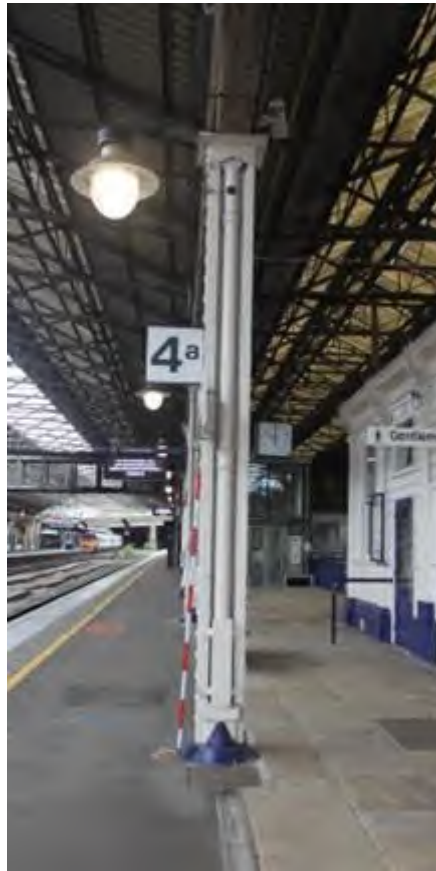
Plate 36: Example of a compound-riveted wrought iron column with 2m scale, facing south
