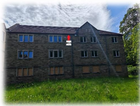
Plate 10: Roost 13 (Building 13, NE. aspect).
