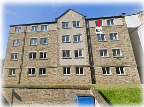
Plate 11: Roost 14 (Building 18, NE. aspect).
