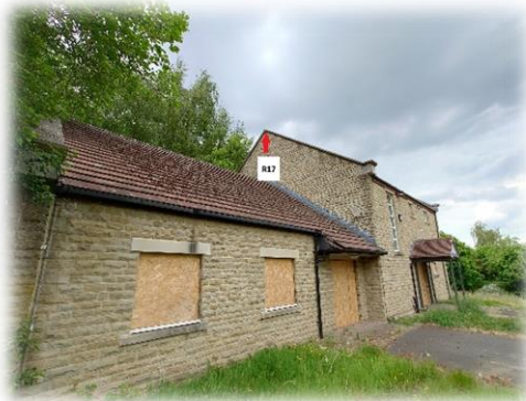
Plate 15: Roost 17 (Building 2, SE. aspect).
