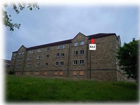
Plate 9: Roost 12 (Building 16, SE. aspect).
