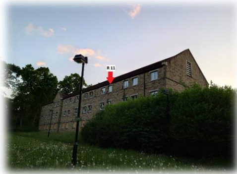
Plate 8: Roost 11 (Building 3, SE. aspect).
