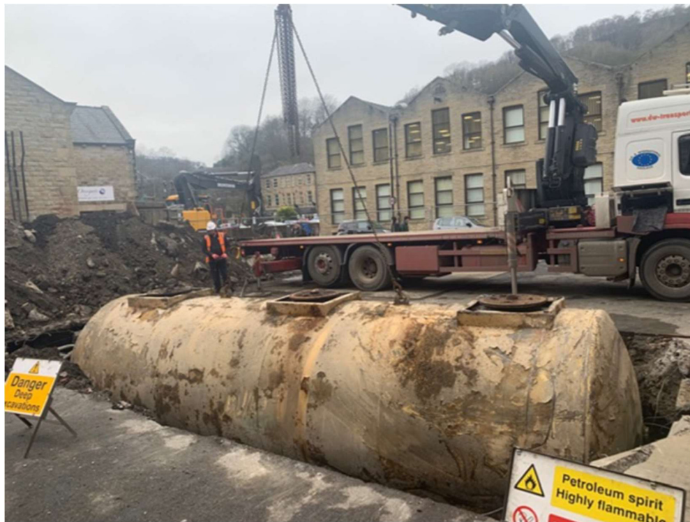
Figure B. The safe removal of a historic tank from the ground after excavation.
