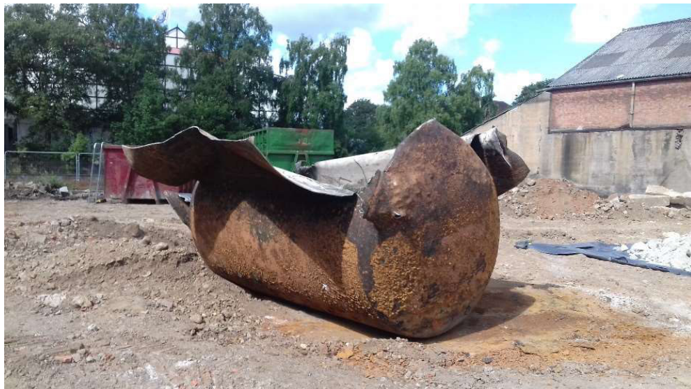
Figure E. Steel tank inspected on the surface after tank pull.
