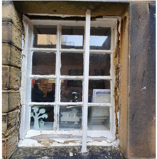
Typical examples of the timber single glazed windows exhibiting multiple defects
