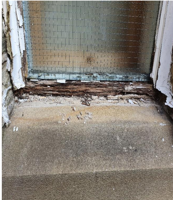
Typical examples of the timber single glazed windows exhibiting multiple defects
