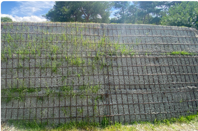
Embankment following hydroseeding
