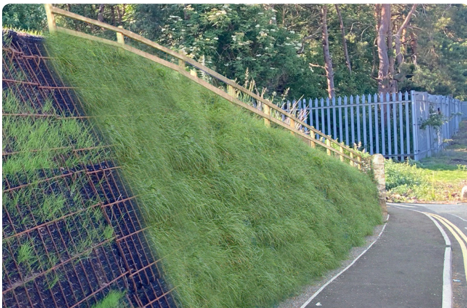
Embankment with hand seeded & hydroseeded areas
