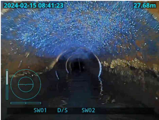
015.jpg, 00:05:16, 27.68 m Point repair, pipe replaced from 9 o'clock to 3 o'clock, Top half replaced
