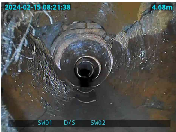
005.jpg, 00:00:45, 4.68 m Point repair, pipe replaced from 10 o'clock to 2 o'clock, Top half replaced
