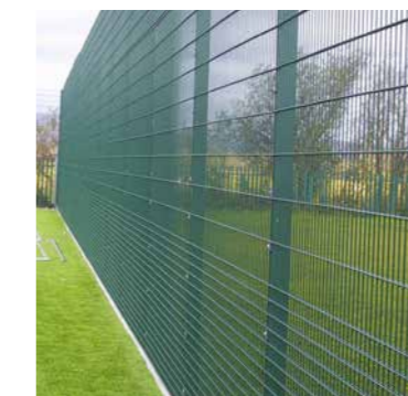
3.0m Rebound Weld Mesh Fencing to MUGA
