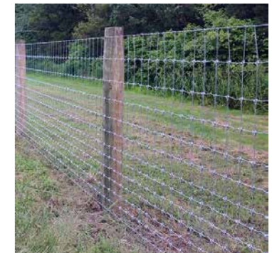
1.5m Galvanised Wire Mesh Fence to Goat's Enclosure
