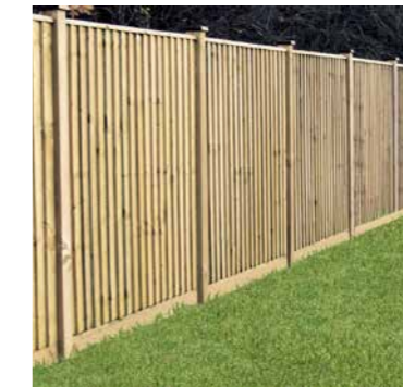
3.0m Vertical Featheredge Closeboard Timber Fencing to Sprinkler Tank
