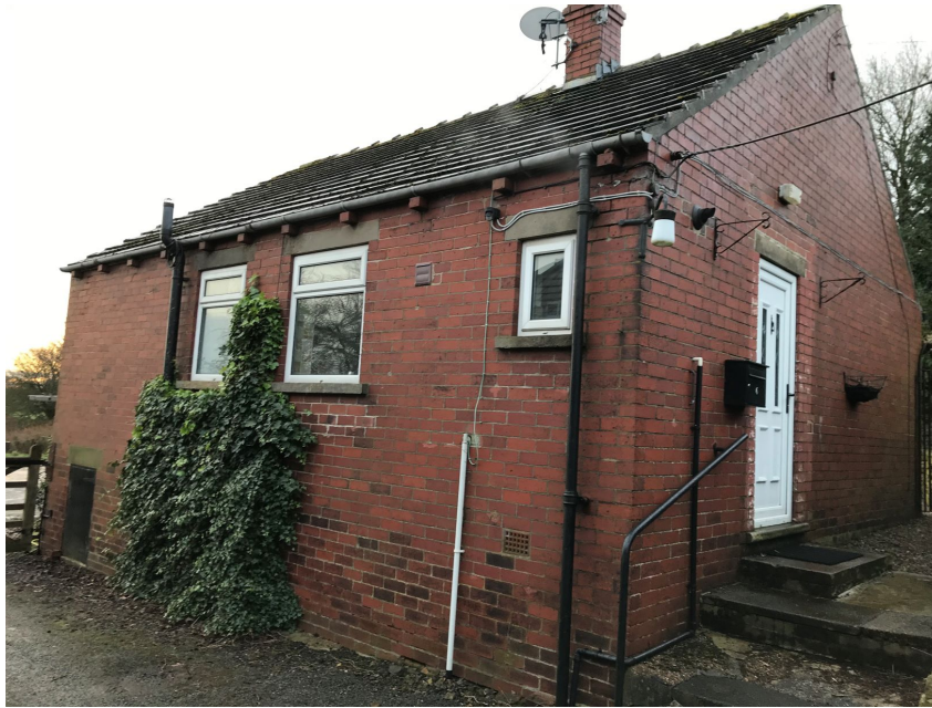
Image 3. - No.4 also elevated from the ground levels.
