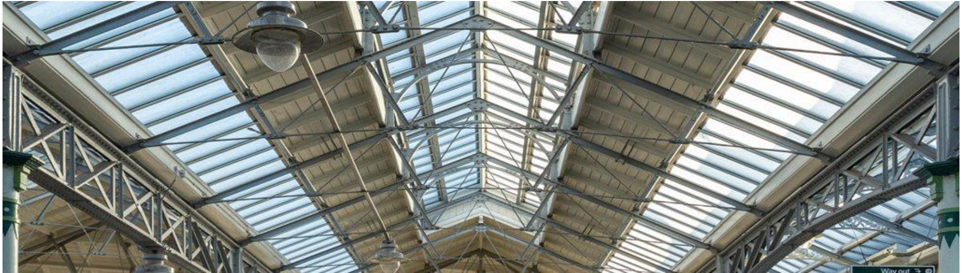
Insert 3 - Roof A Glazing: Example of Georgian Wired Polycarbonate Rooflight Glazing (Twinfix, Lewes Station roof).
