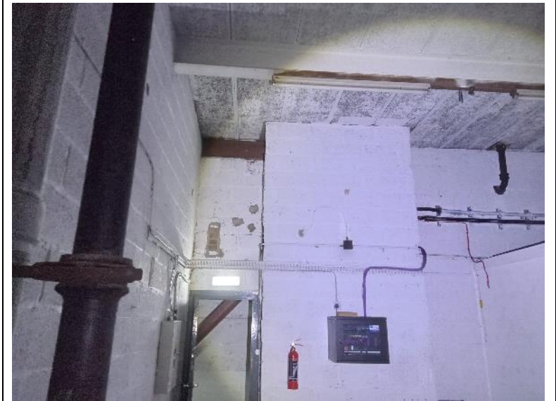
Figure 23. Roof space 2 – well sealed.
