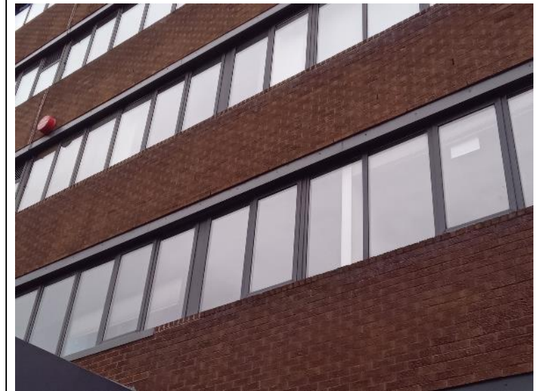
Figure 7. Easten elevation – supporting walls intact.
