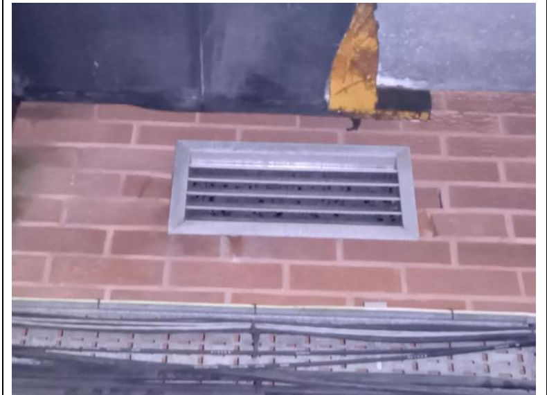
Figure 11. Western elevation – sealed vent.
