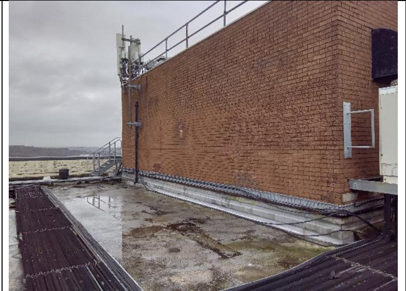
Figure 16. Supporting walls intact.
