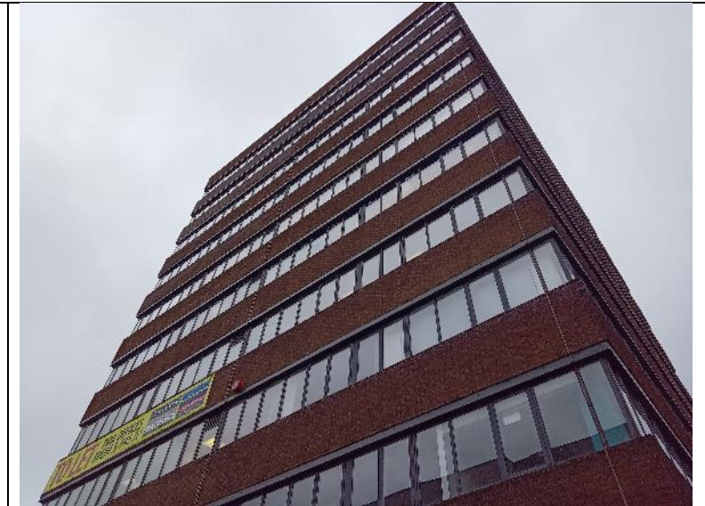
Figure 6. B1 – facing the eastern elevation.
