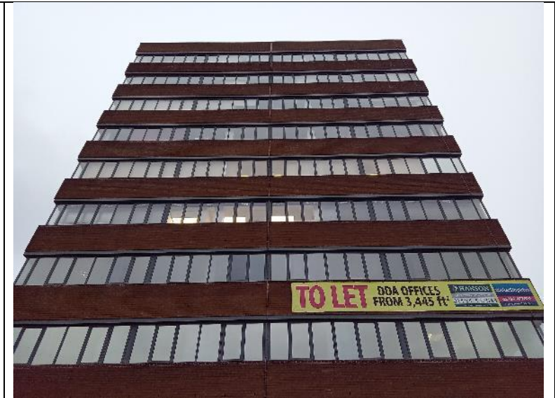
Figure 12. B1 – facing the southern elevation.
