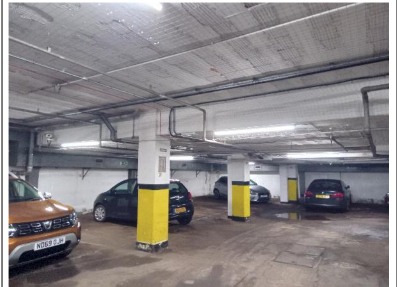
Figure 27. Basement – well lit car park.
