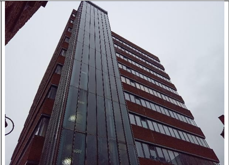
Figure 10. B1 – facing the western elevation.
