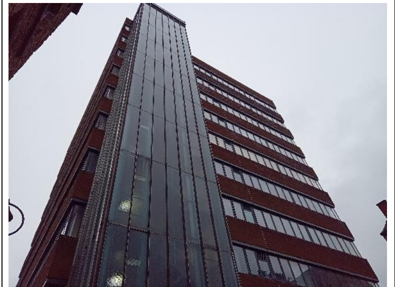
Figure 10. B1 – facing the western elevation.
