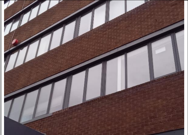
Figure 7. Easten elevation – supporting walls intact.
