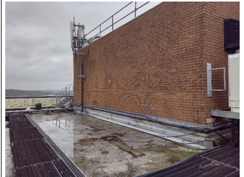
Figure 16. Supporting walls intact.
