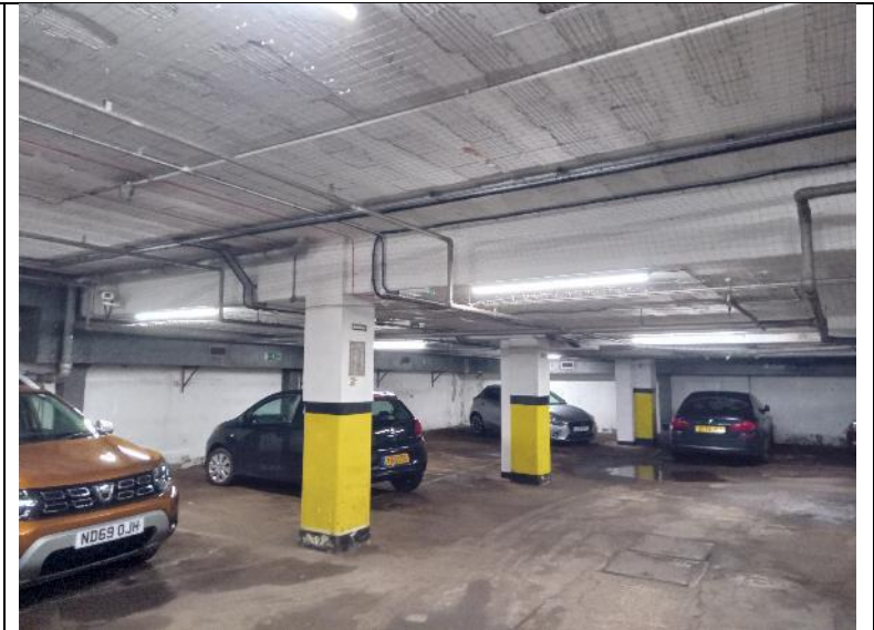
Figure 27. Basement – well lit car park.
