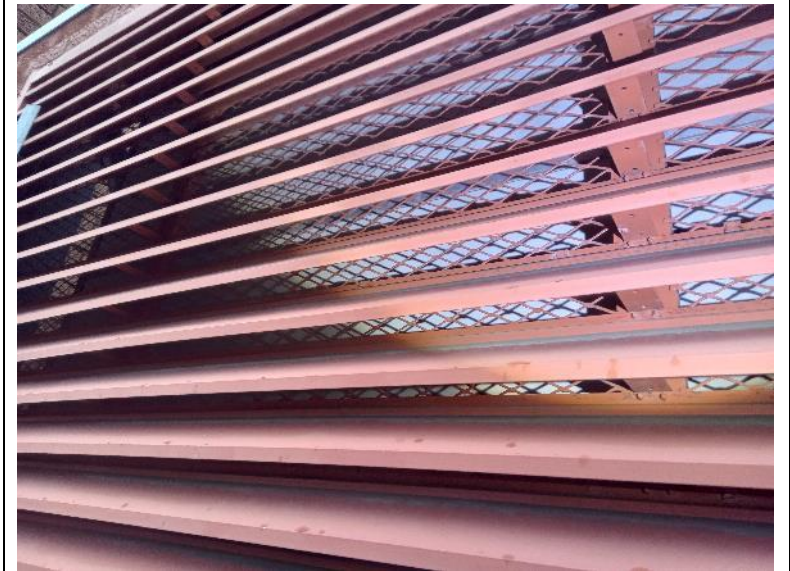
Figure 14. Southern elevation – vent.
