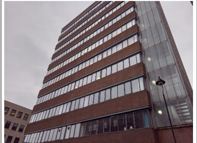
Figure 8. B1 – facing the northern elevation.
