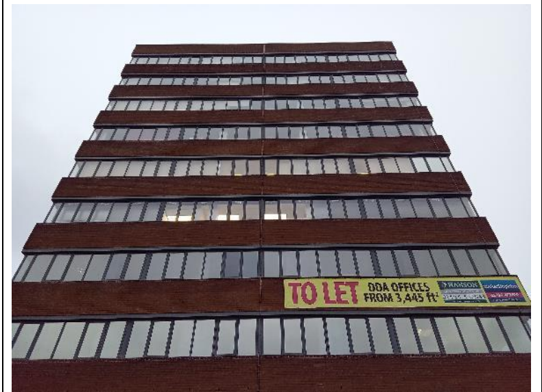
Figure 12. B1 – facing the southern elevation.
