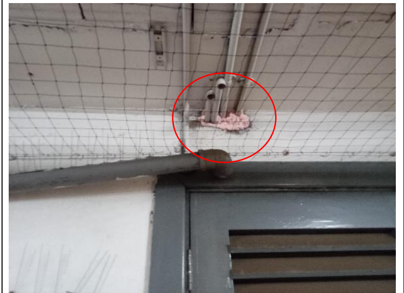
Figure 28. Basement – supporting wall crevices infilled.
