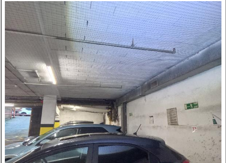
Figure 30. Basement – majority of ceiling intact.
