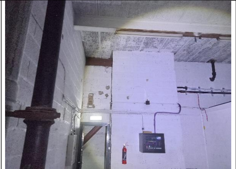
Figure 23. Roof space 2 – well sealed.
