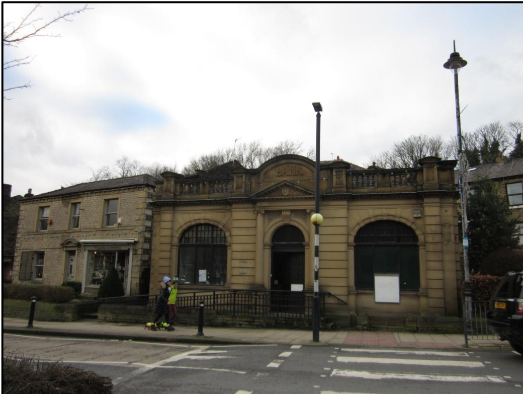
Photograph 1. Location of the proposed restaurant within the former Lloyds Bank building
