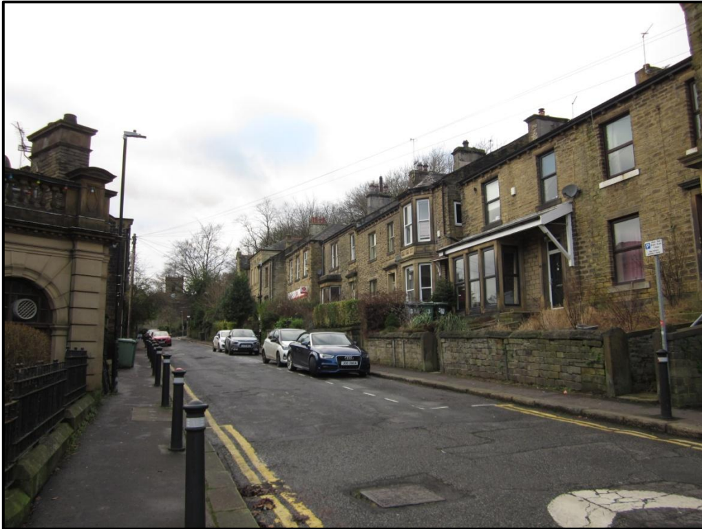
Photograph 2. Existing residential properties on Lewisham Road
