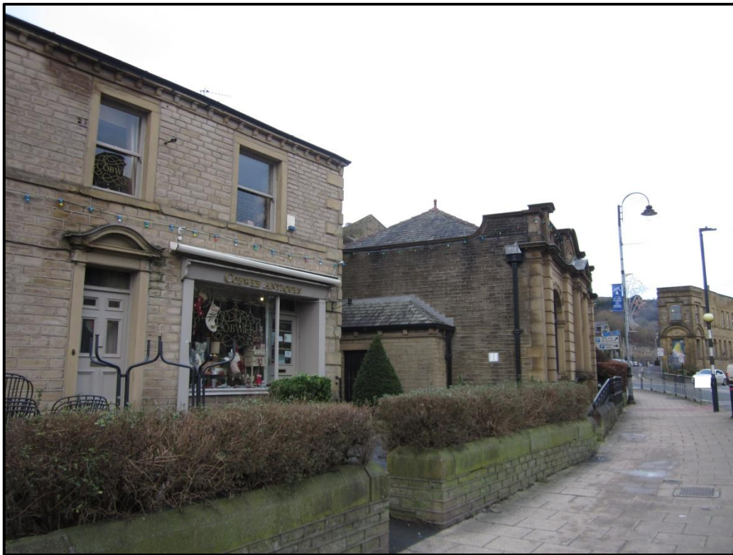
Photograph 6. Commercial premises to the West of the proposed restaurant on Carr Lane
