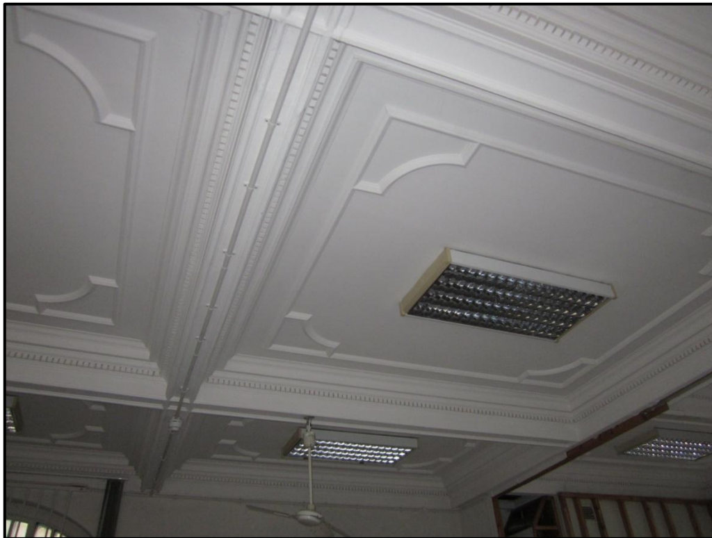
Photograph 7. Existing ornate lath and plaster ceiling
