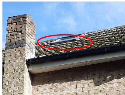
Image 04: Lifted tiles either side of Velux window
