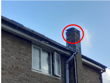
Image 01: Worn brickwork on chimney
