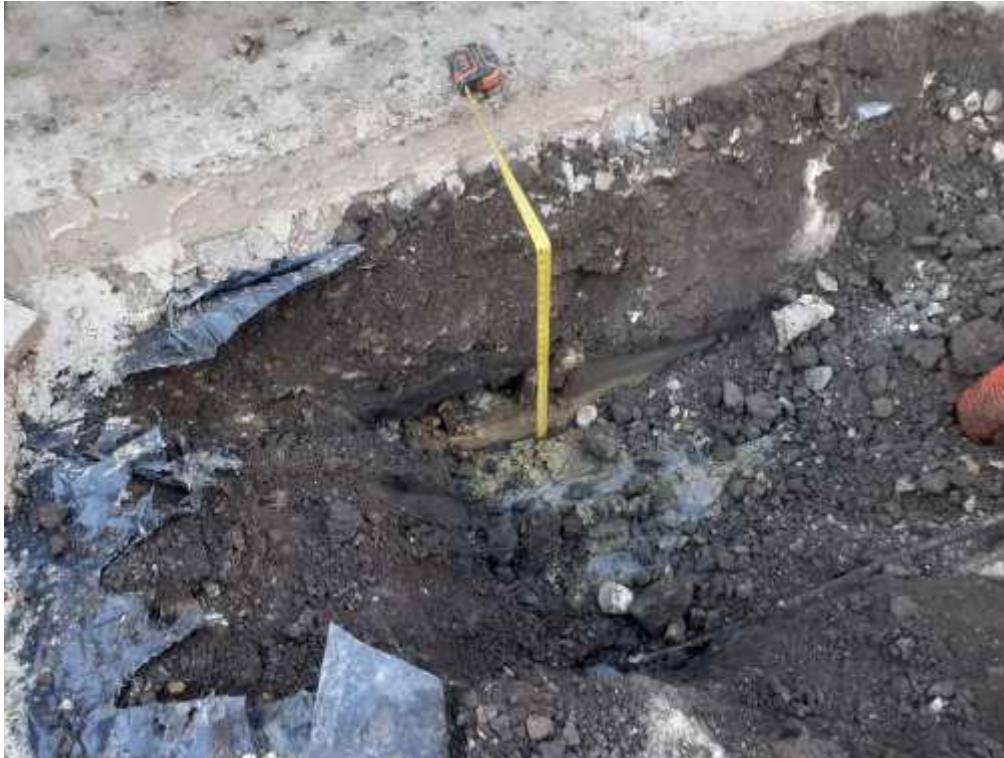
Plate 3: Picture of completed trial pit
