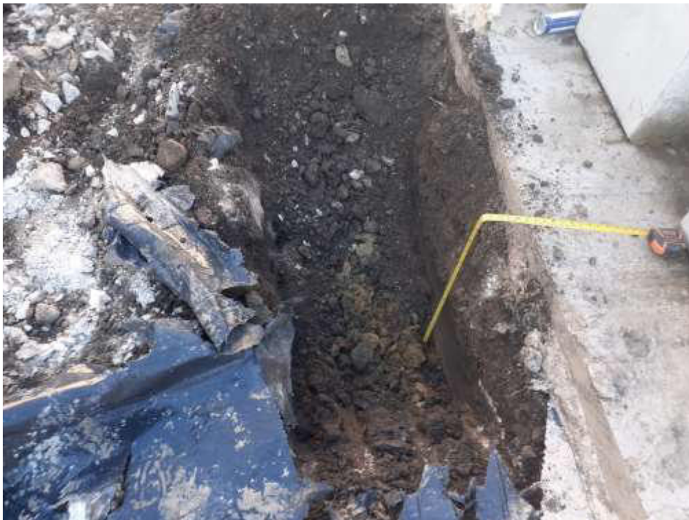
Plate 4: Picture of completed trial pit
