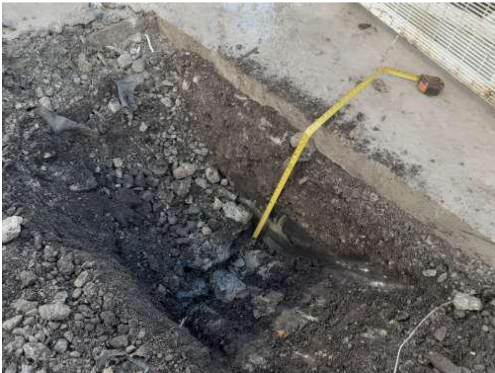
Plate 2: Picture of completed trial Pit
