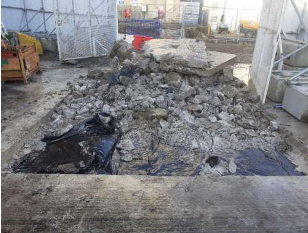
Plate 5: Trial pit area constrained by hoarding and adjacent building
